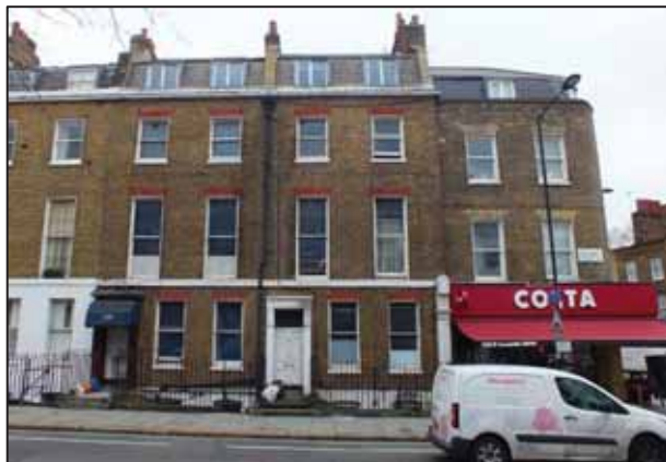
Photo 1: Front façade of Nos. 109 (left) and 110 (right) Guilford Street, looking northwest
