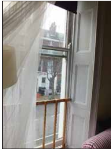
Photo 8: Wooden panelling in window reveal in No. 110: first floor, front bedroom
