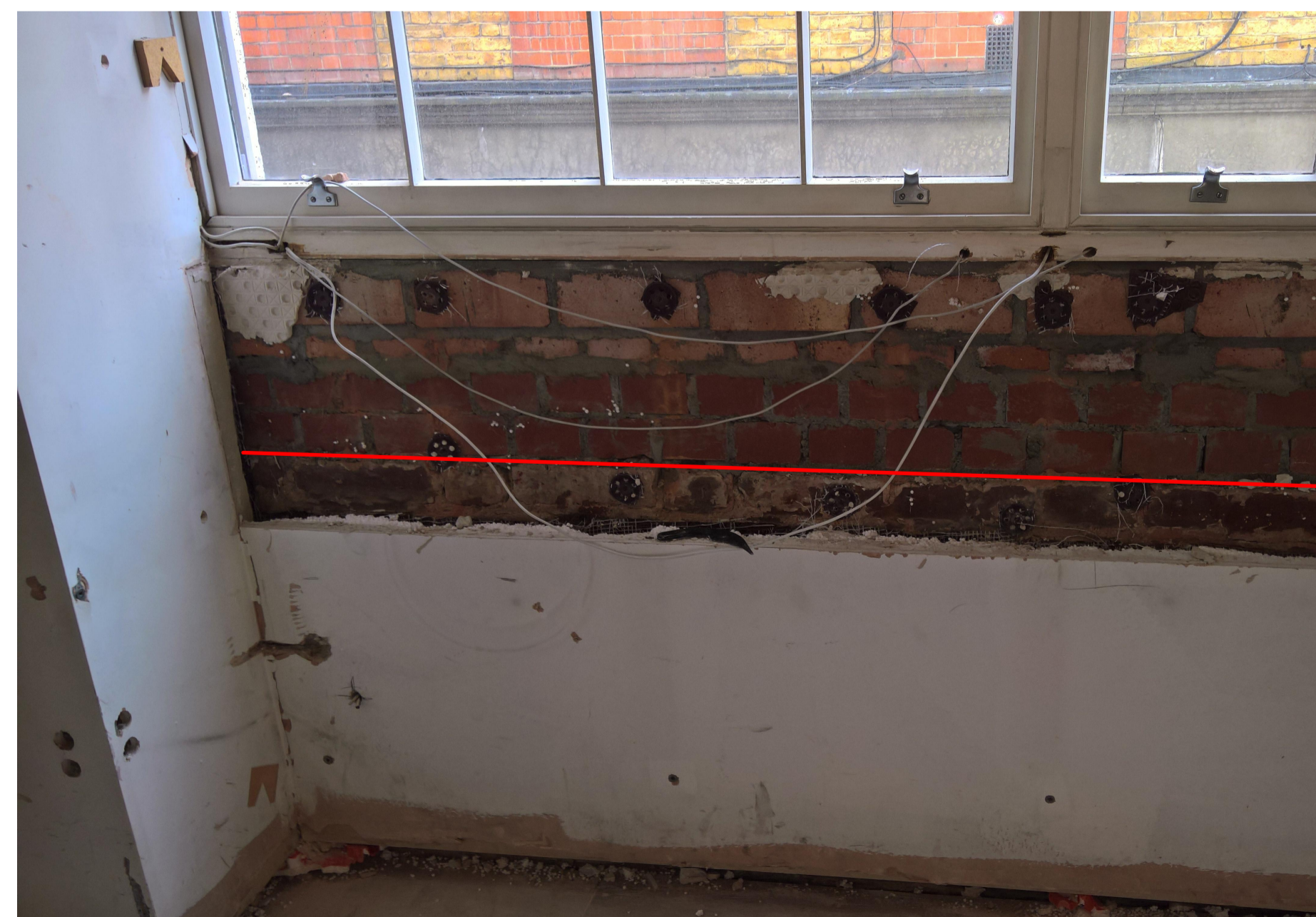
2 Investigation photos of Existing First Floor Windows showing 300mm of new brick infill to reduce the opening size
