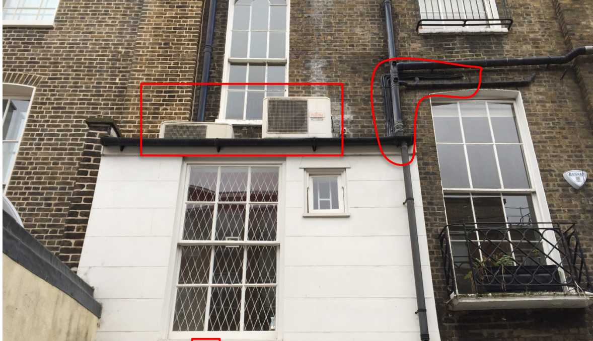
Above and Left: Existing unsightly AC units and feeds located on rear façade are to be removed (outlined in red)
