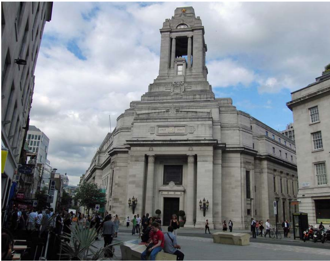
Figure 1: View of western tower looking along Great Queen Street
