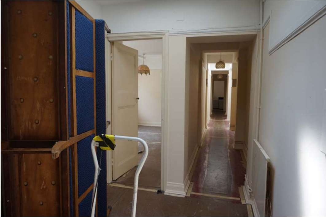
Figure 9: Internal corridor within apartment
