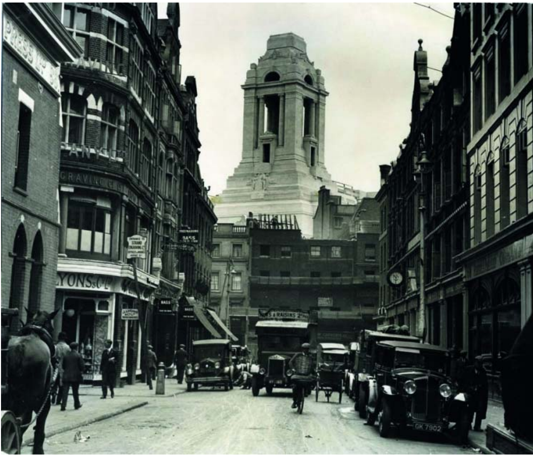
Figure 7: View over partially demolished buildings 1931 (©UGLE)
