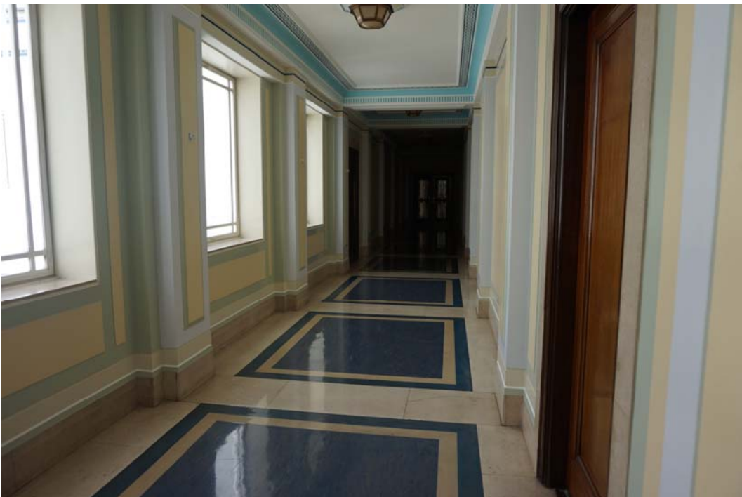
Figure 8: Access corridor outside third floor apartment
