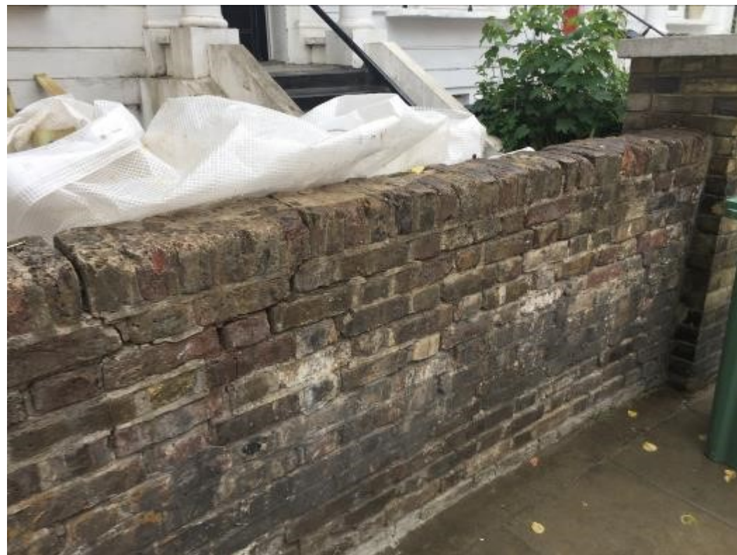
PHOTOS OF EXISTING FRONT BOUNDARY WALL. THE WALL HAS STRUCTURALLY FAILED AND IS CRACKED & LEANING.
