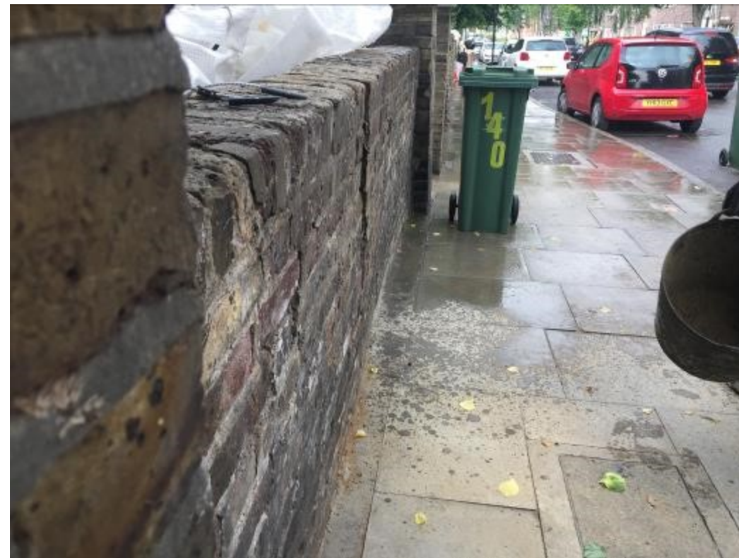
PHOTOS OF EXISTING FRONT BOUNDARY WALL. THE WALL HAS STRUCTURALLY FAILED AND IS CRACKED & LEANING.
