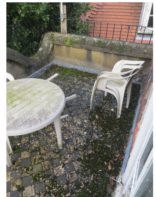
Photograph of existing terrace condition
