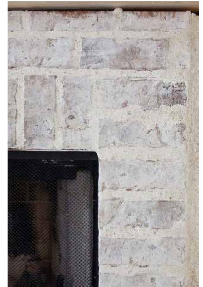
Mortar washed brickwall
