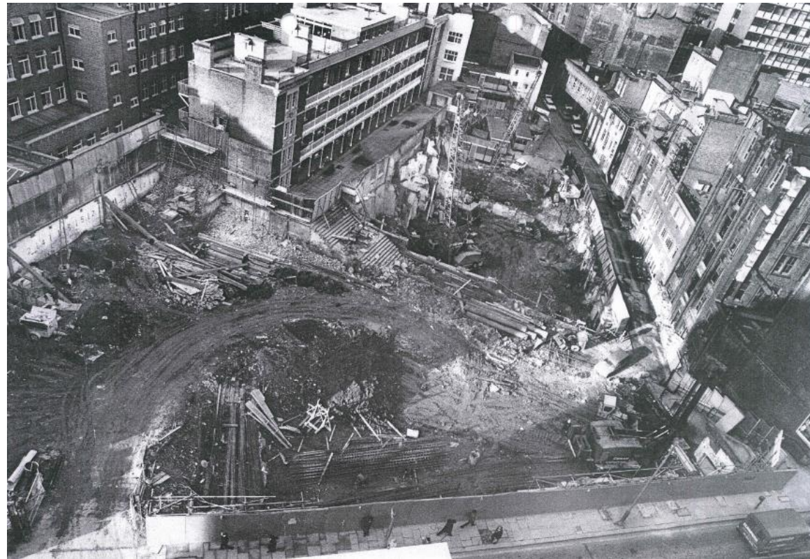
Figure 9: Photograph taken during basement excavation for 1979 development
