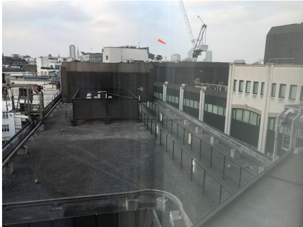
Figure 7: View of Saffron Hill block roof plant enclosures
