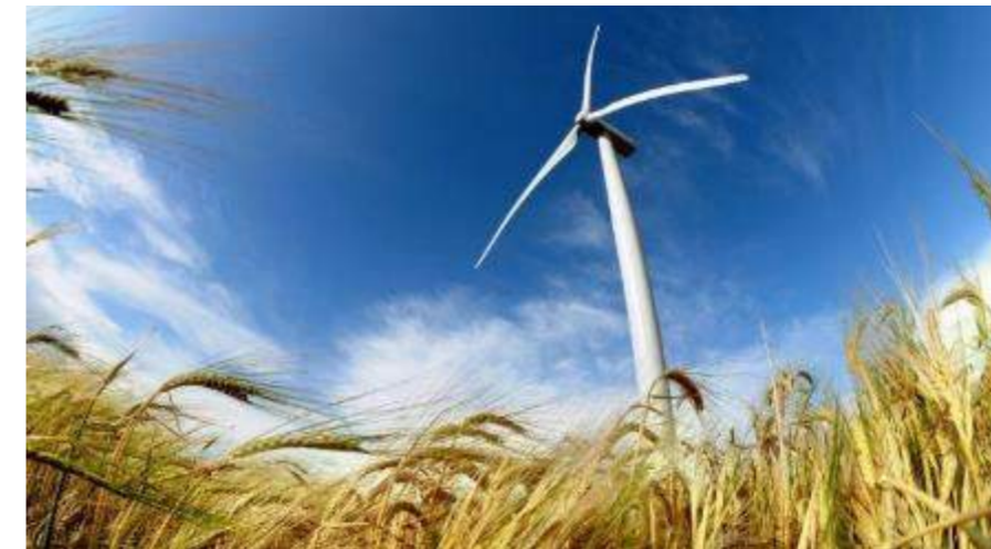
Figure 23. Image of a wind turbine
