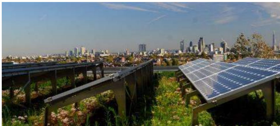
Figure 12. Indicative PV / green roof arrangement
