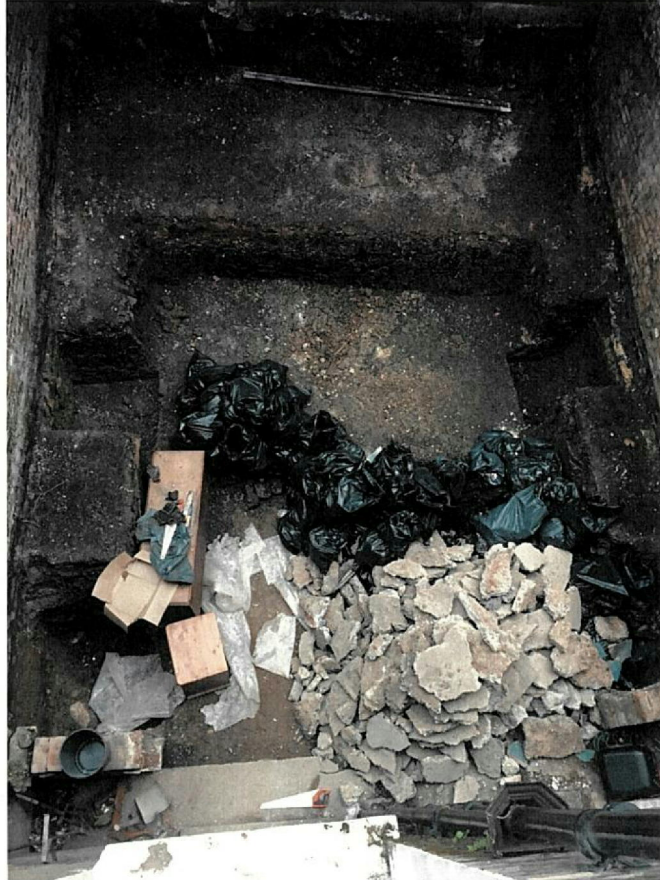
Fig 1 - foundations in rear garden, photo from 30 April 2017
