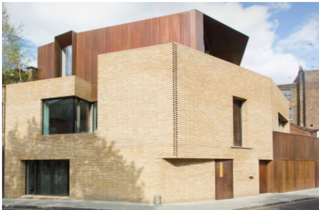
a) building selected by the architect as an example of bronze cladding with beige brick; b) Close-up of varying shades of bronze.
