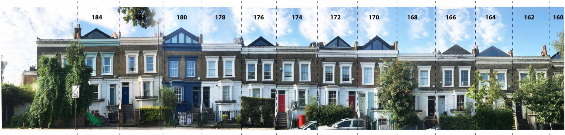
View of the terrace from the street.
