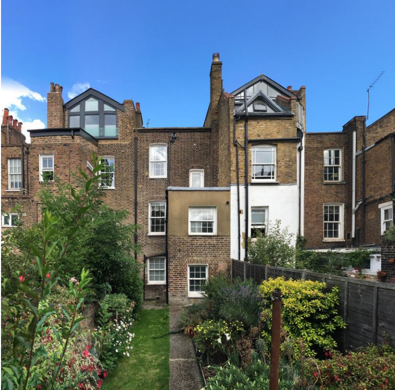
Existing rear view of the house
