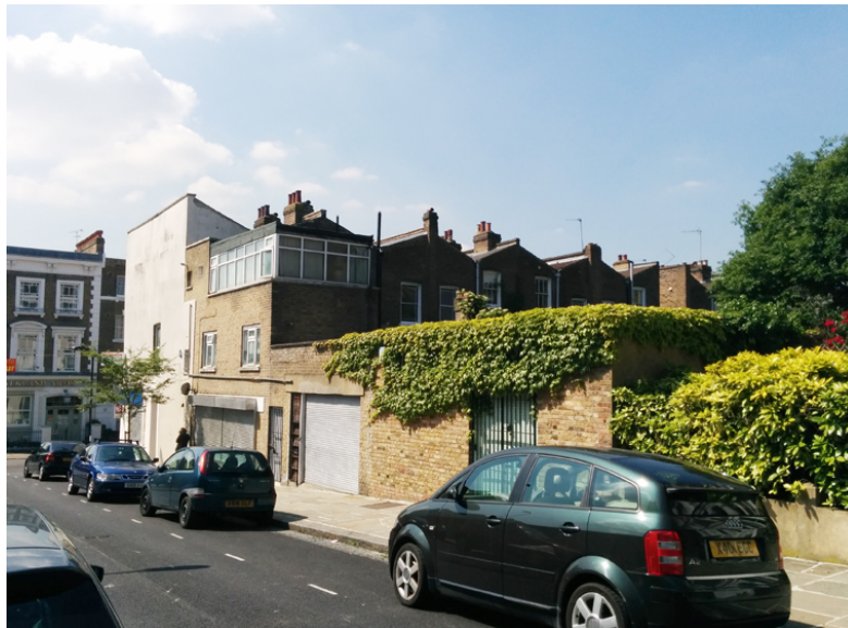
Front and side view from Falkland Road and Montpelier Grove
