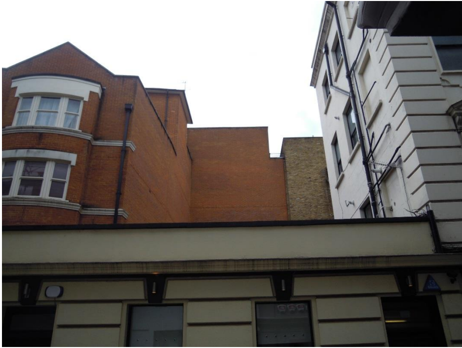
neighbouring flank walls at rear of site
