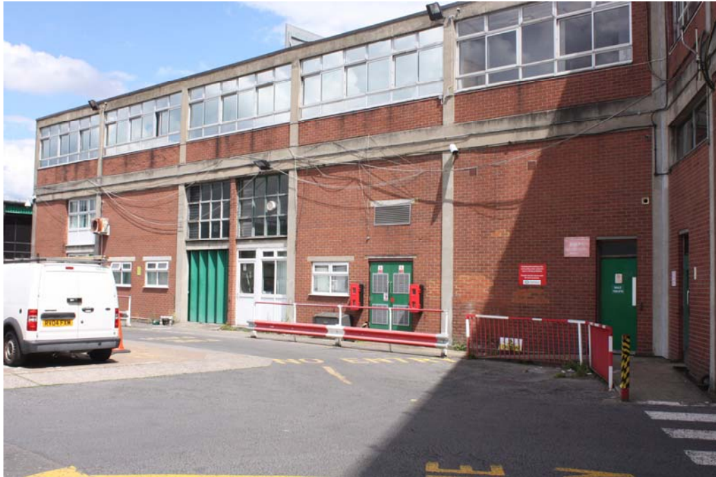
Internal Elevation of east side
