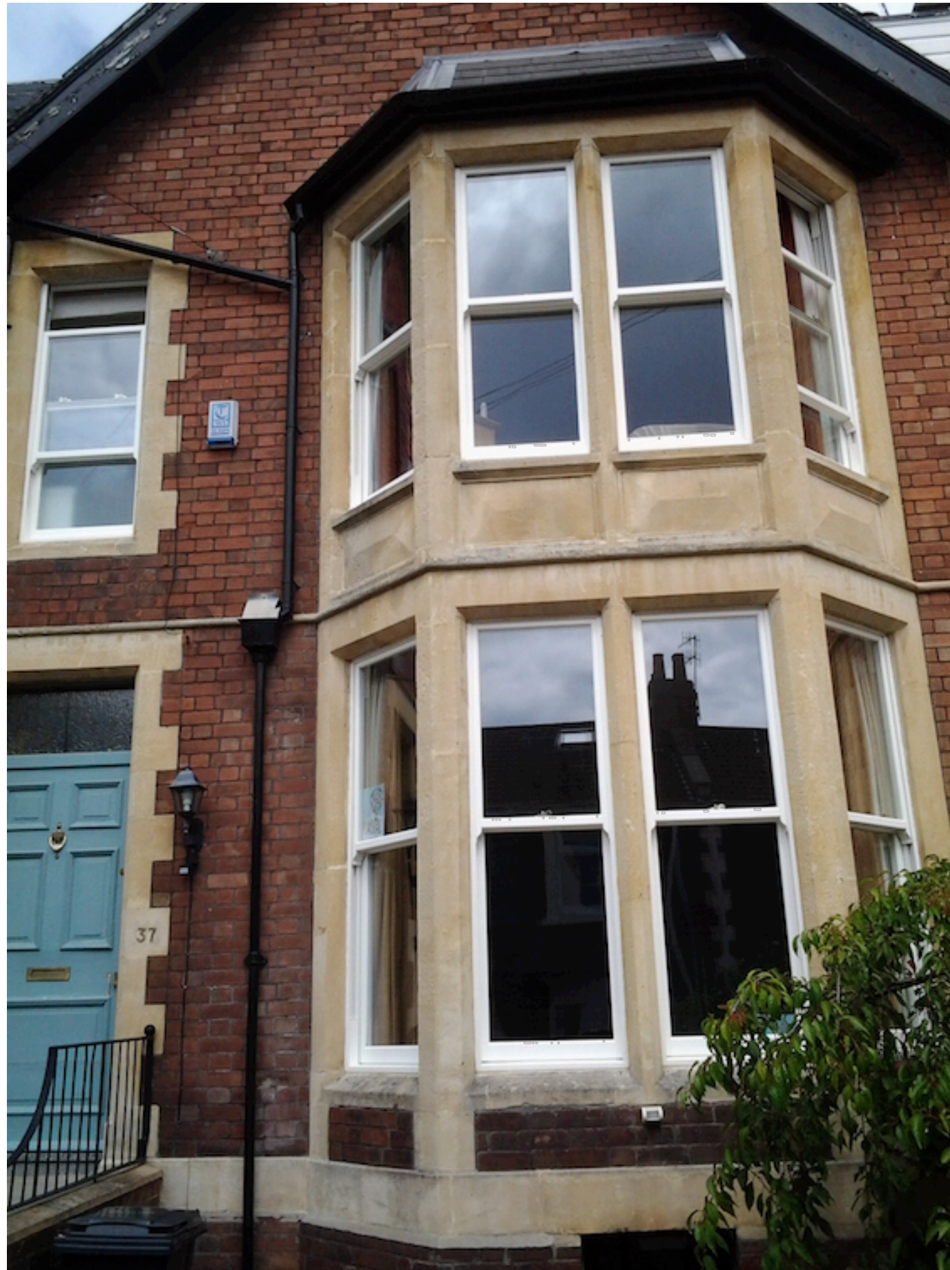
Photo of Typical Proposed Replacement Windows
