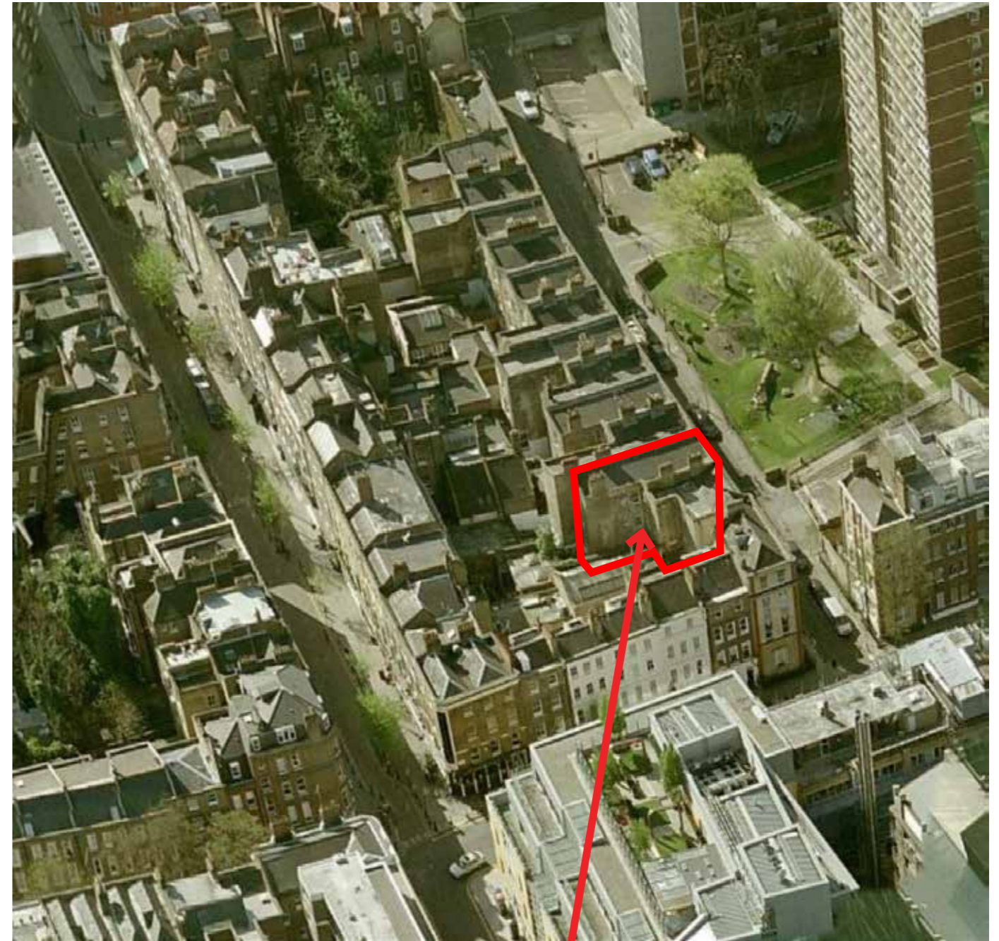
FLAT 24 A - GROUND FLOOR AND LOWER GROUND FLOOR OF 24-26 ORDE HALL STREET
