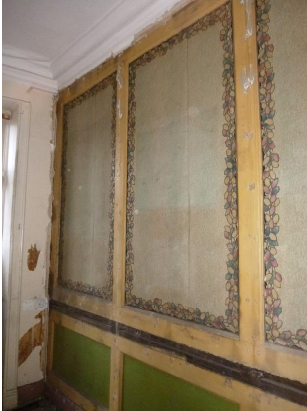
Figure 2: West wall, viewed facing south
