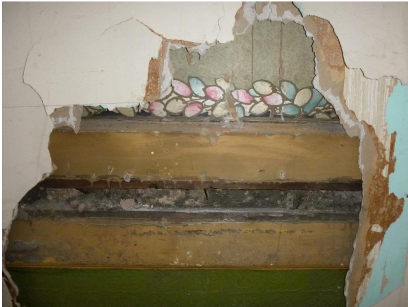
Figure 5: East wall, viewed facing east
