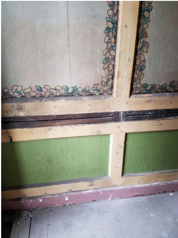
Figure 3: West wall, viewed facing east
