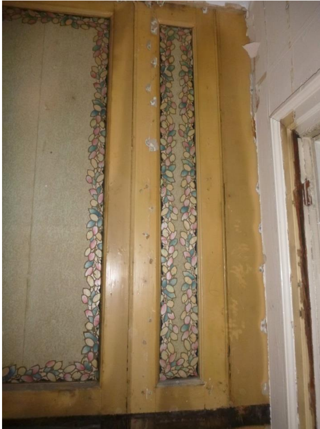
Figure 4: West wall (northern end), viewed facing west
