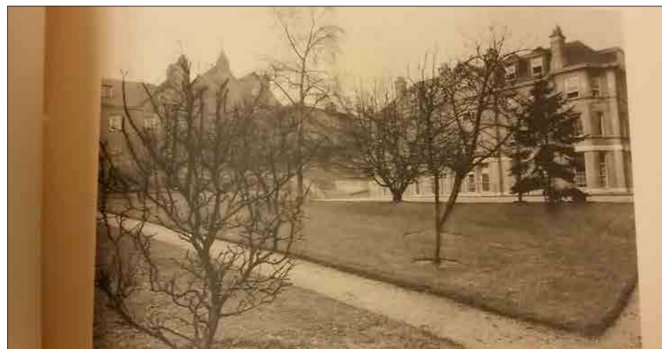
Eastern Quadrangle looking toward Maynard wing and Lady Chapman Hall
