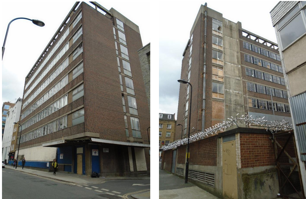
Figures 1 & 2: The Site, viewed from Tottenham Street (figure 1) and Tottenham Mews (figure 2)
