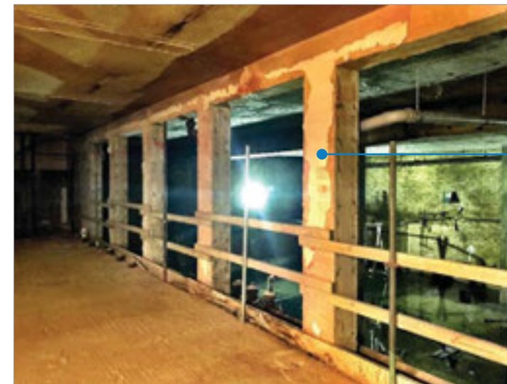
3.02 Existing columns below Ground Floor at northern elevation of existing building.
