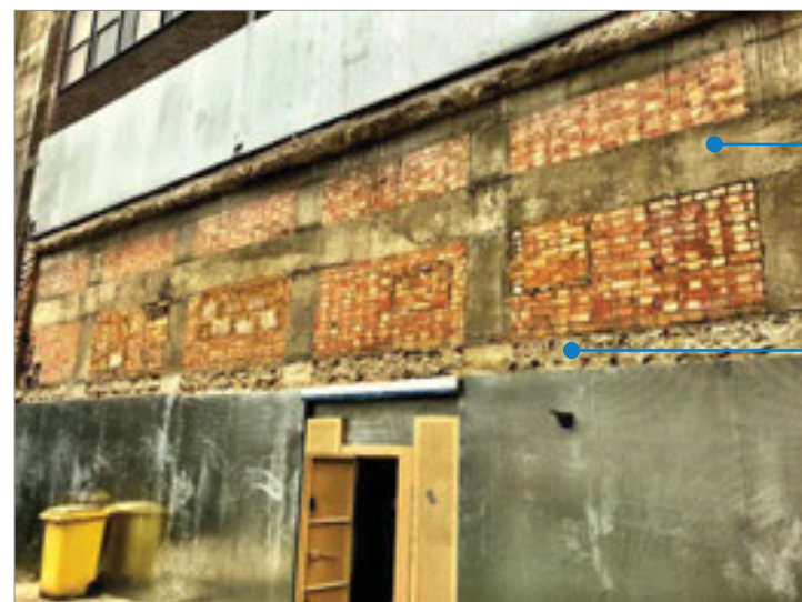
2.10 External face of north elevation of the building above Ground Floor.
