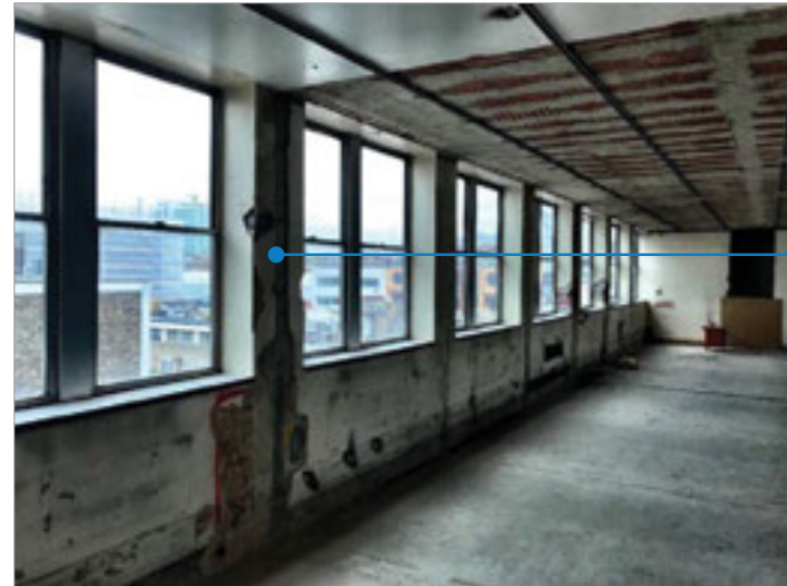
2.09 Existing column line on north elevation of building.
