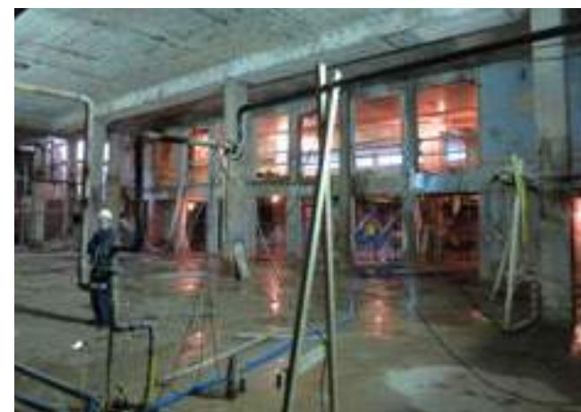
Existing double height basement (looking south)
