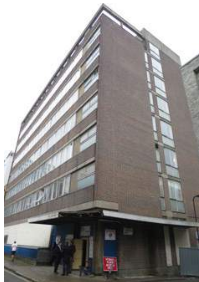
Existing Front Facade
