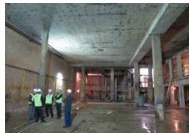
Existing double height basement (looking east)
