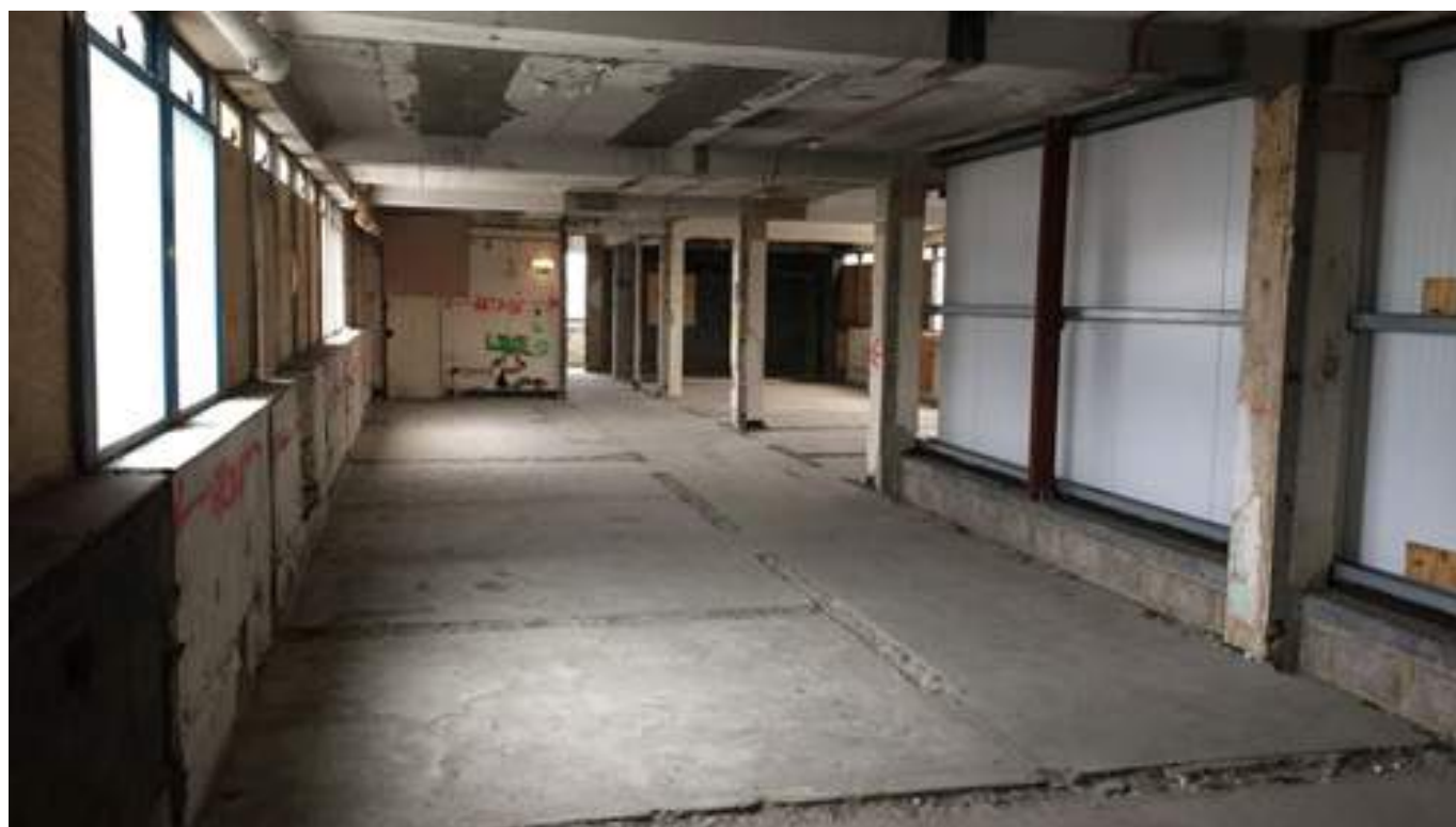
Existing AAC concrete slabs at roof level
