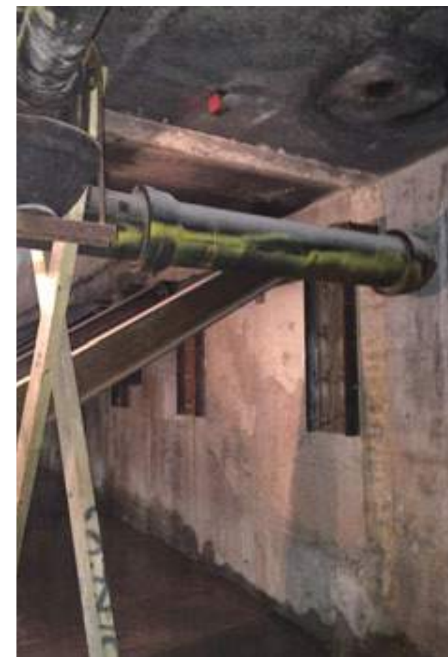
Existing Drainage Outlet at High Level Basement
