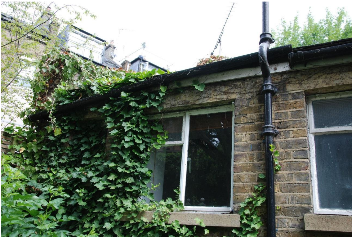
Photograph 2: Roof and rainwater goods to rear
