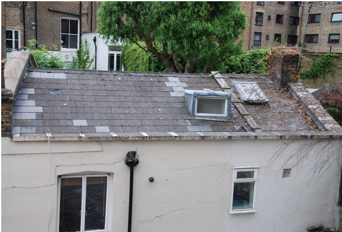
Photograph 1: Main roof from front
