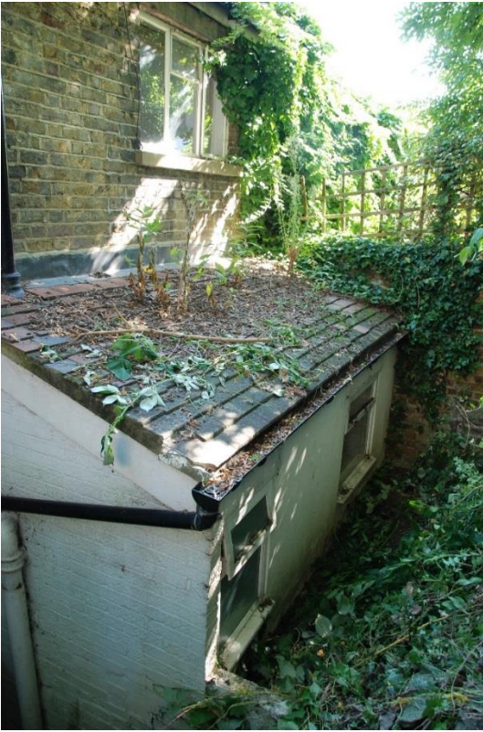
Photographs 3&4: Roof to rear addition and detail showing cracked tiles and rotten fascia board
