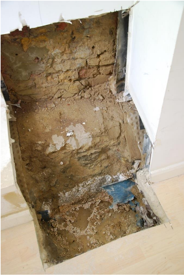
Photographs 8&9: Damp membrane/drylining and trapped moisture at slab level
