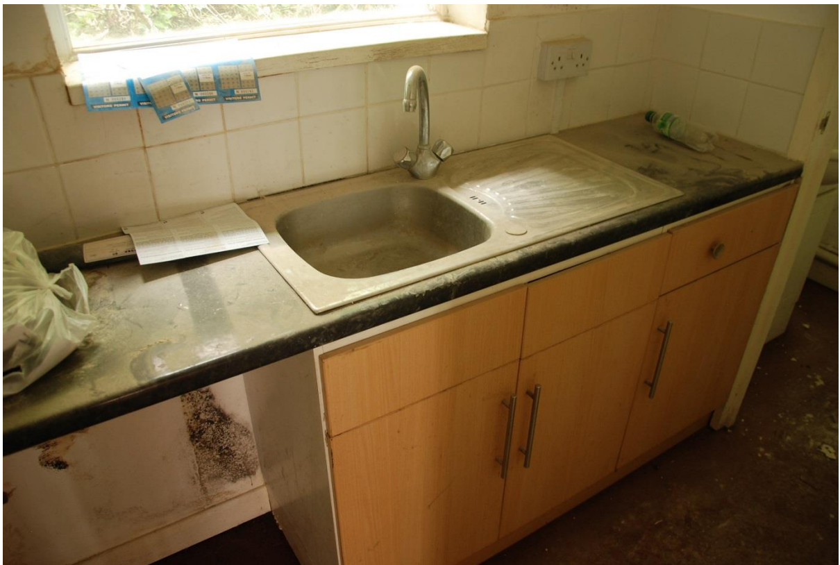
Photographs 14 & 15: Internal kitchenette
