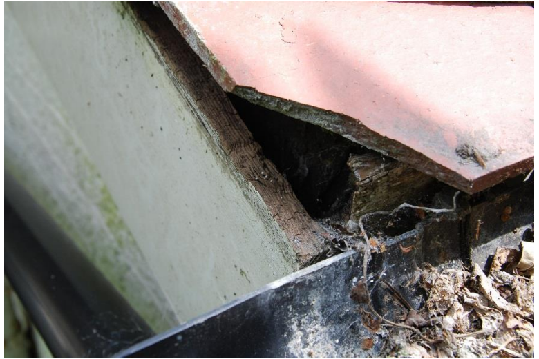
Photographs 3&4: Roof to rear addition and detail showing cracked tiles and rotten fascia board
