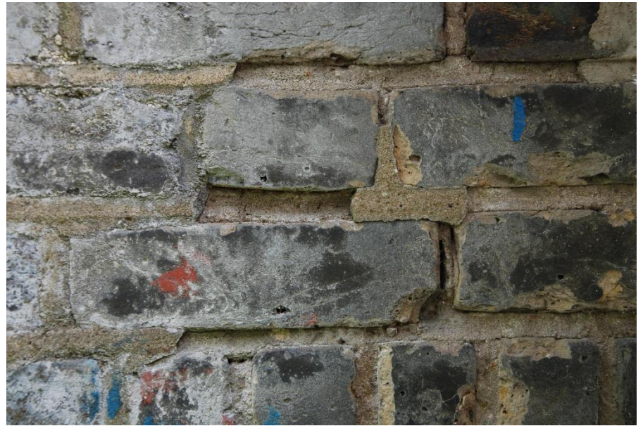
Photograph 6: Detail of brickwork to rear elevation
