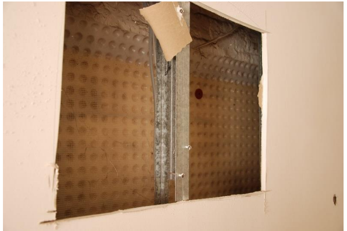
Photographs 8&9: Damp membrane/drylining and trapped moisture at slab level
