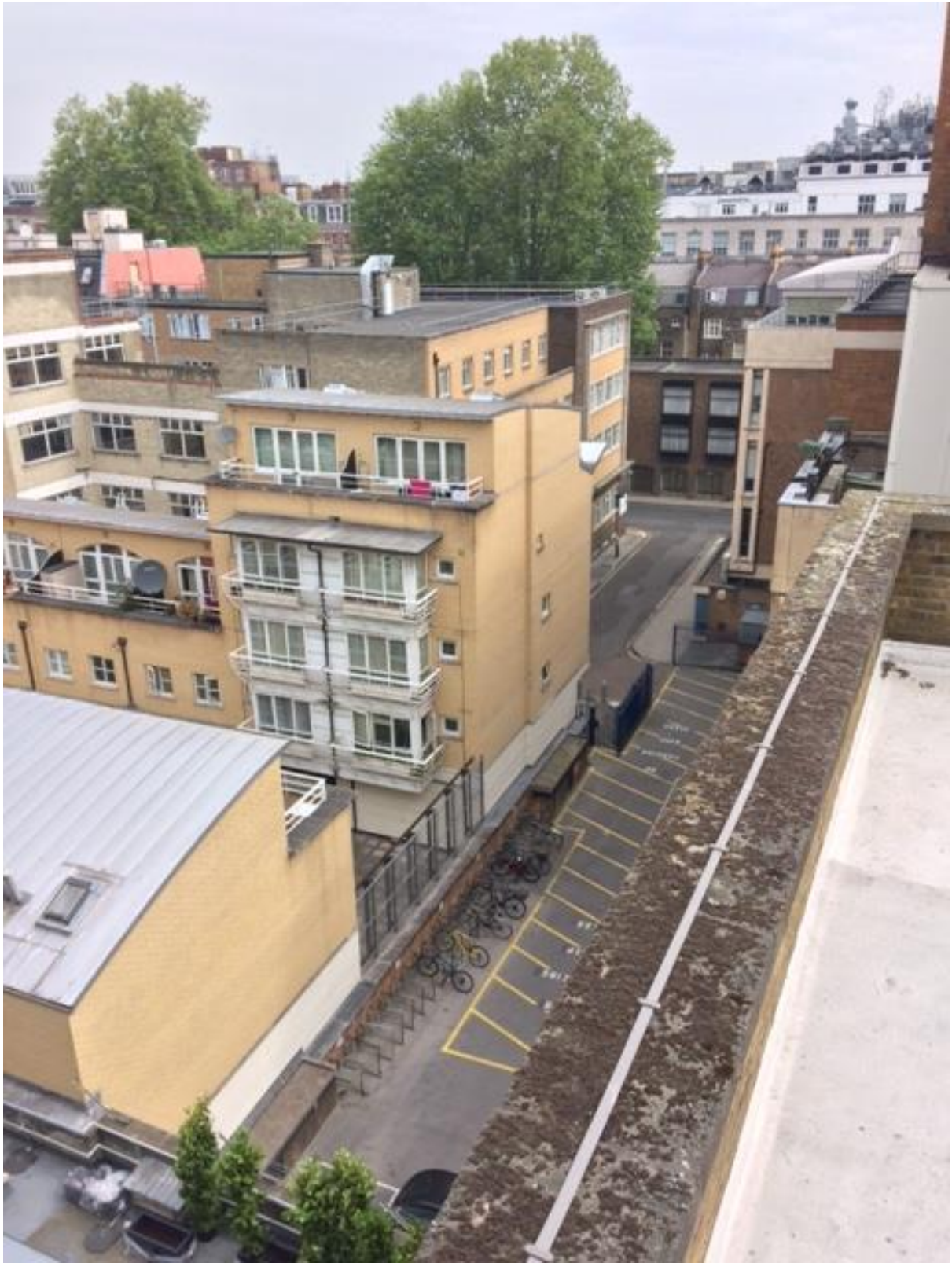
Photo 4 - Residential flats to the rear (Rossetti Court)
