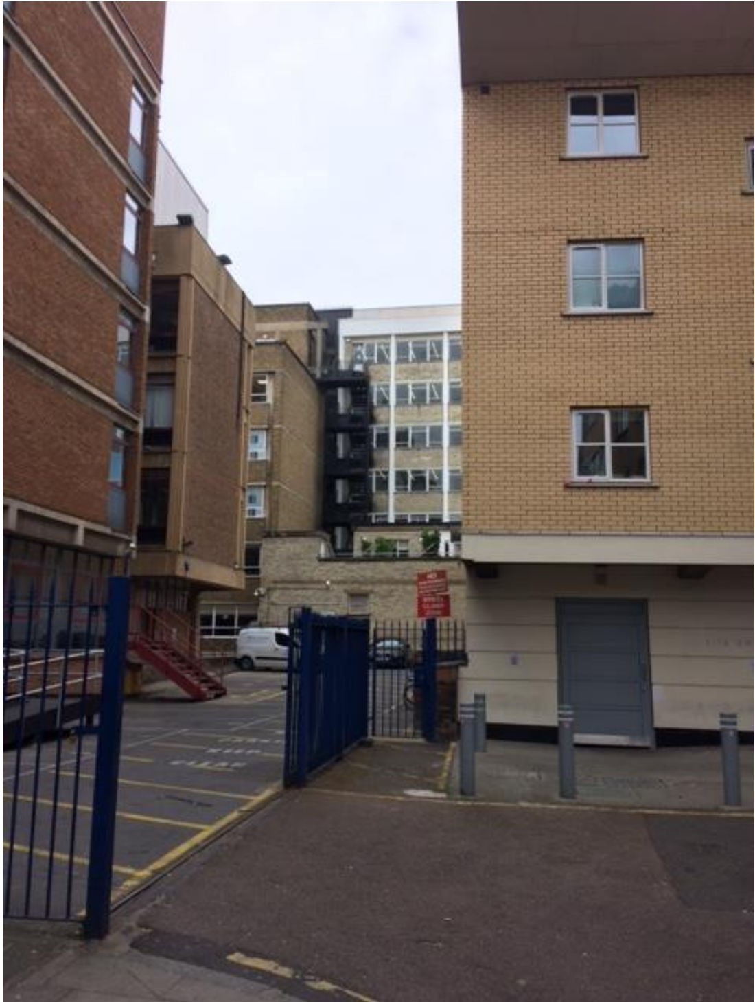
Photo 1 - Rear Elevation from Ridgmount Place
