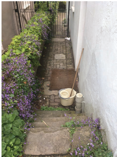
Range of side step treatments, finishes and gradients along Provost Road, therefore the original is impossible to determine nor is there a common situation able to follow in the sake of continuity.
