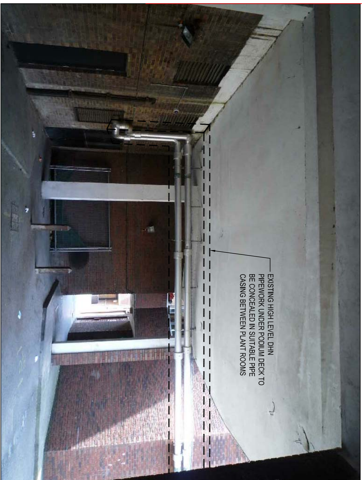
ALTERNATIVE DETAIL FOR REPLACEMENT HTG GAS & BOWS PIPES AVOIDING TRENCHING IN ENTRANCE AREA
