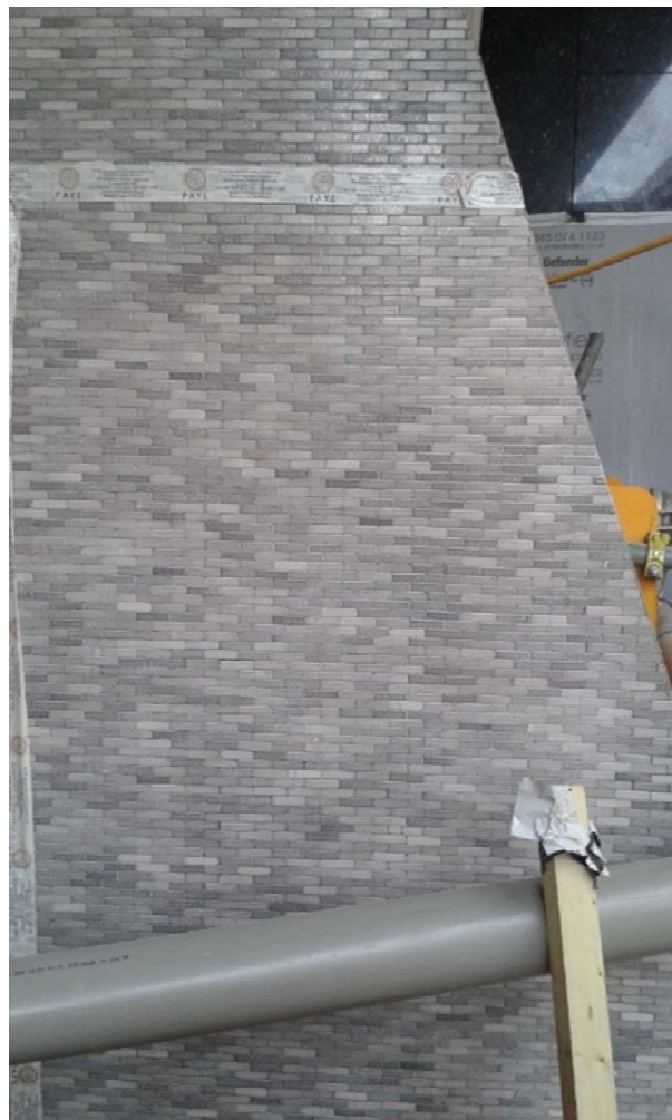
Photo 2. Type 1 - Repair sample
