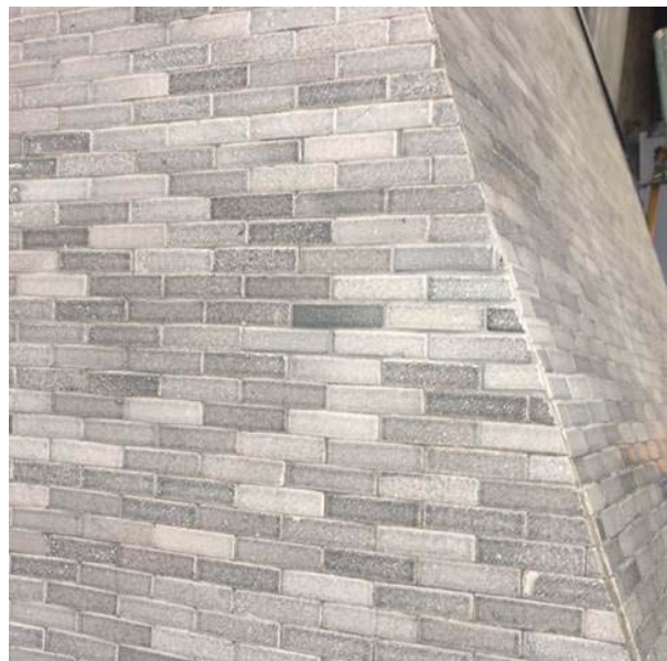
Photo 1. Type 1 - Repair sample
