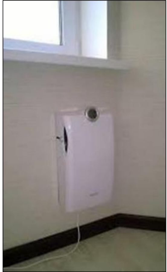
Figure 2: Examples of Internal Acoustic Ventilation system.
