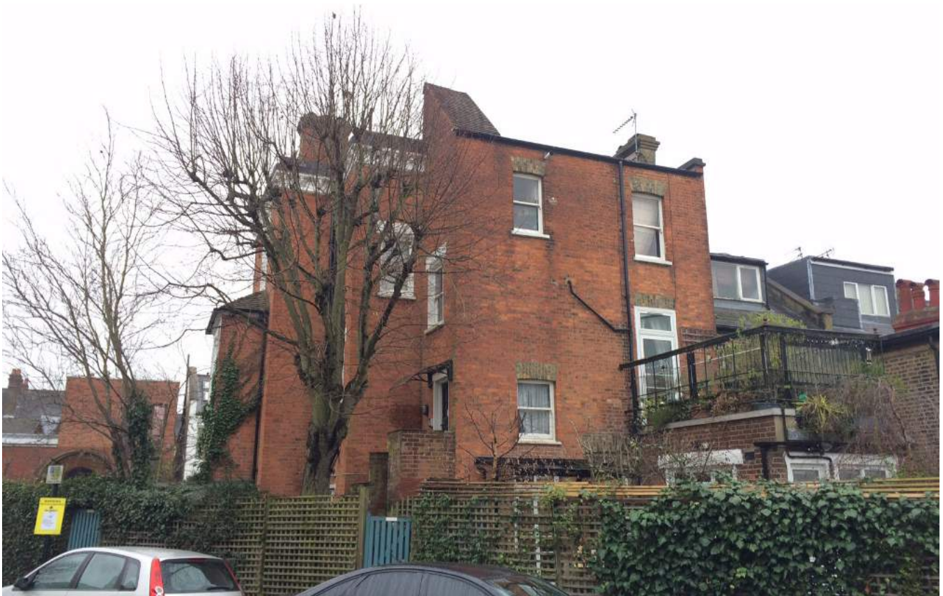
Rear elevation to 57 Burrard Road as viewed from Ingham Road, showing the existing roof access stair housed in a remnant of the original tiled roof volume and brick gable wall.
