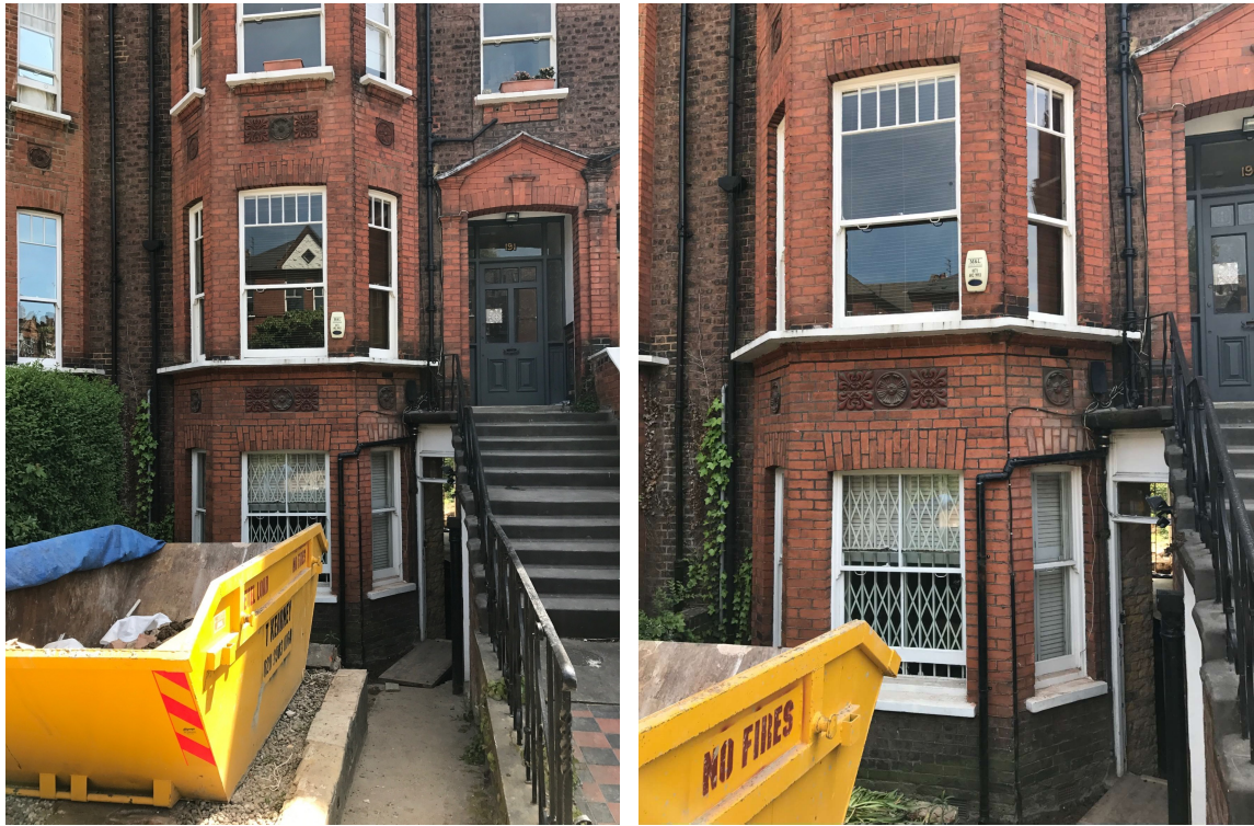
Photos of front elevation, showing windows.
