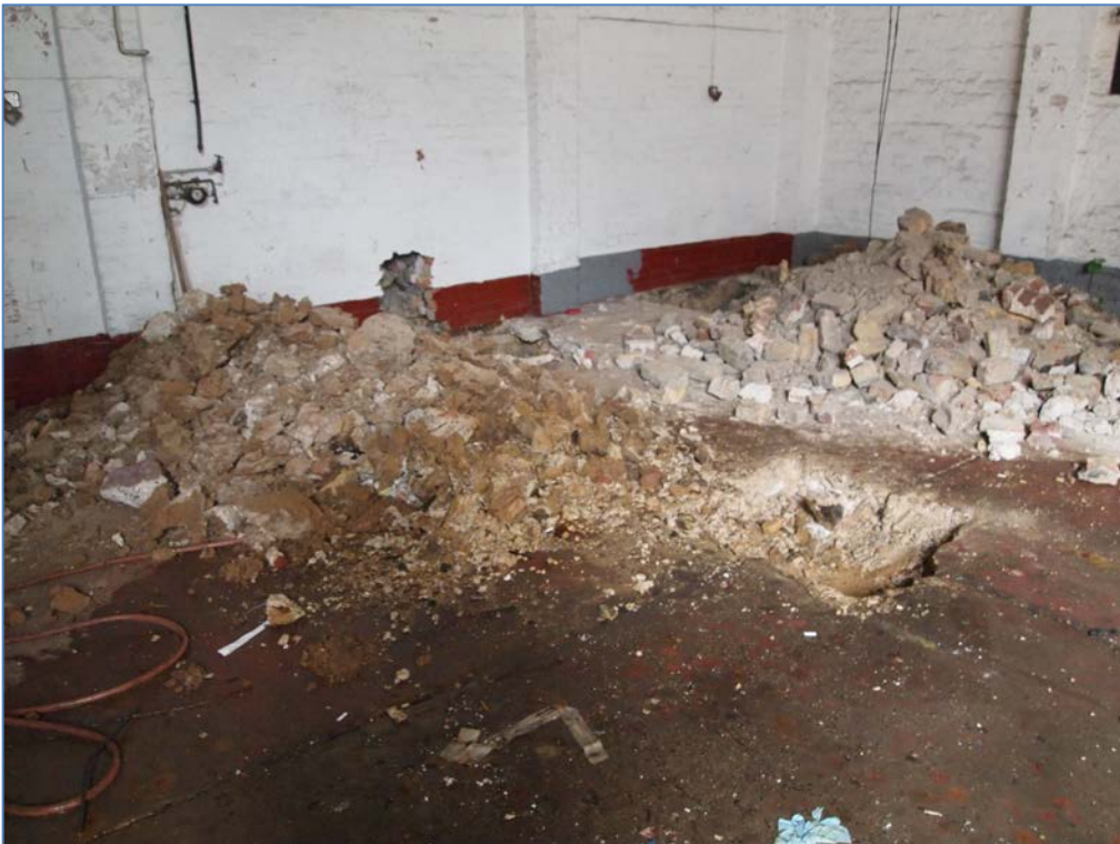
Trial Pits in Main Workshop.
