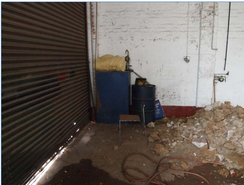
Waste Oil Tank against south-western boundary wall.
