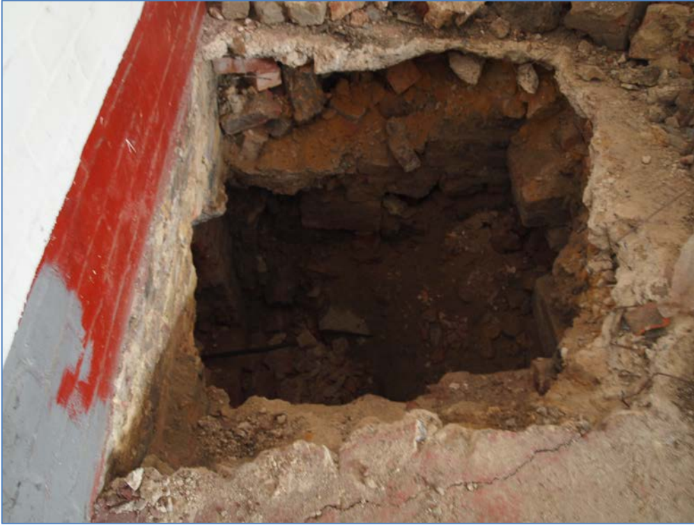
Trial Pit in Main Workshop.
