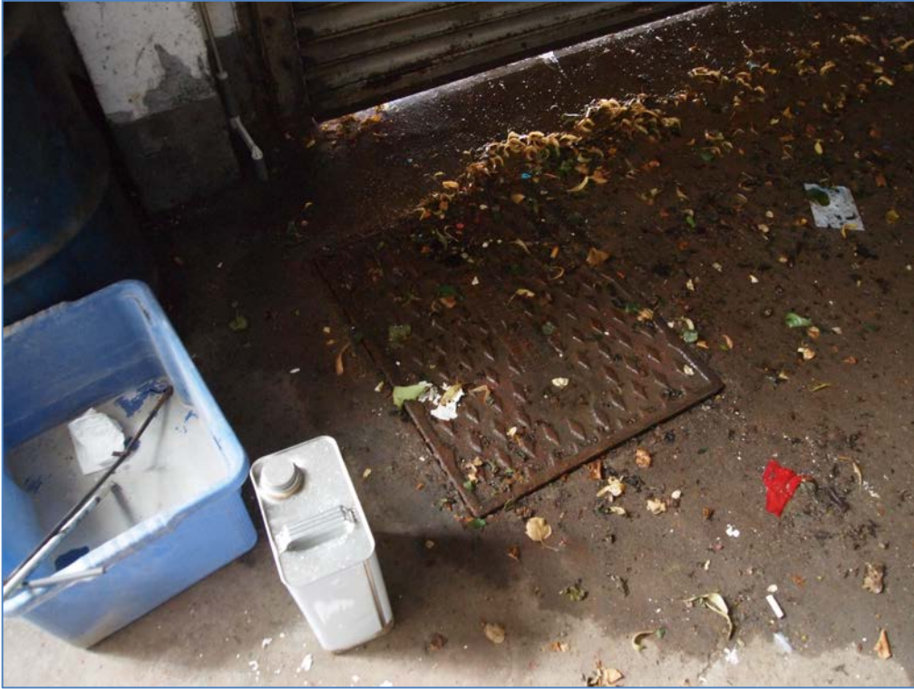
Existing Inspection Chamber in Main Workshop.
