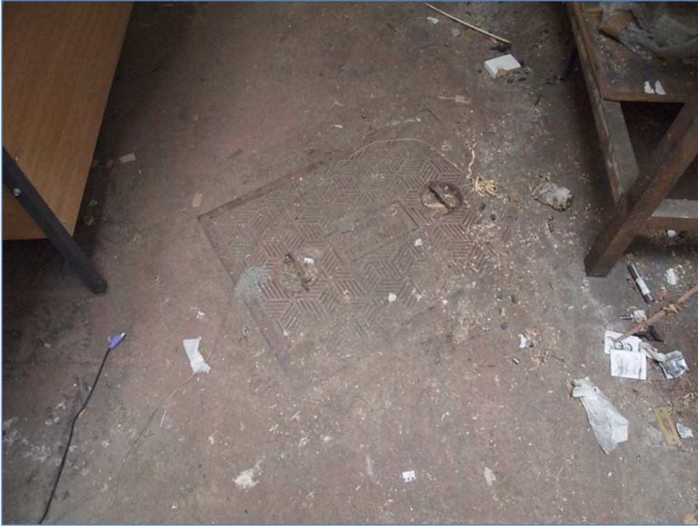
Inspection Chamber in Smaller Workshop.
