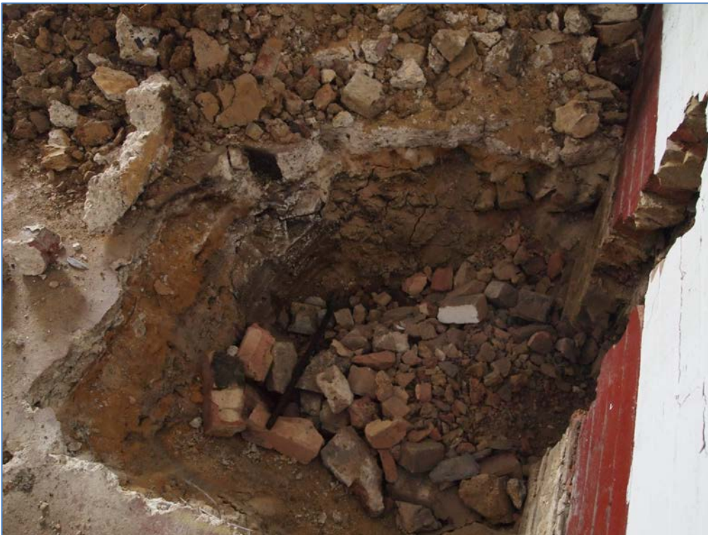
Trial Pit in Main Workshop.
