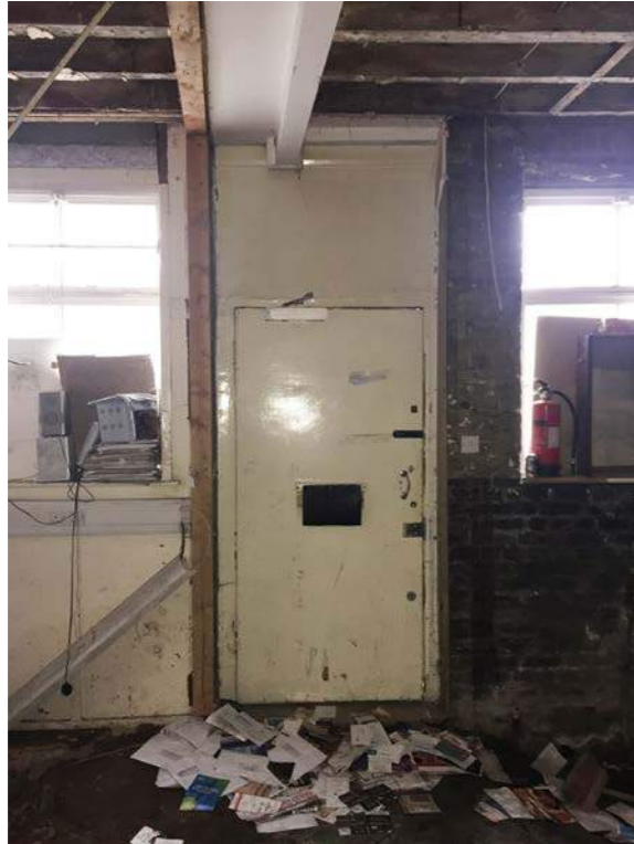
1. Inside view of front facade door
