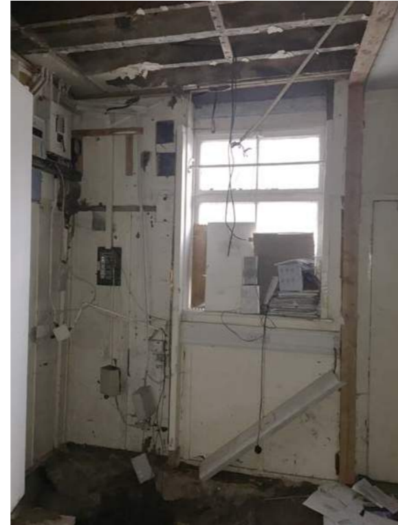
2. Inside view of front facade window
