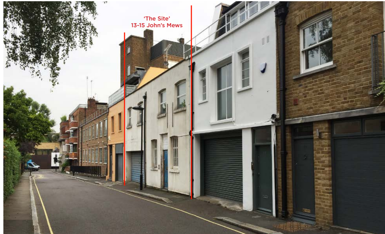
01 - Front elevation looking North on John's Mews
