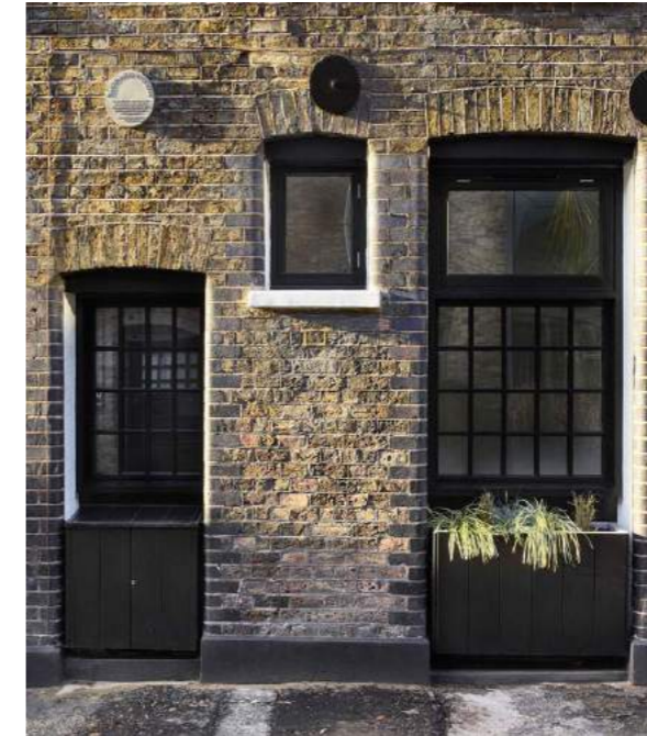
Fig.04 - Doughty Mews/Roz Barr Architects
