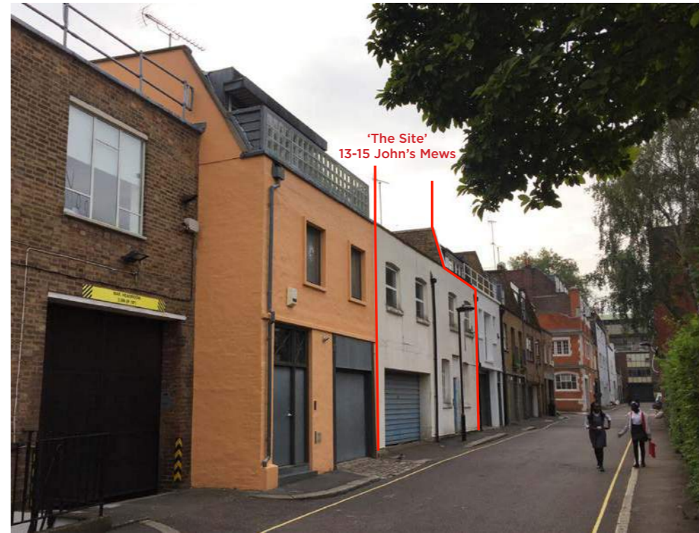
02 - Front elevation looking South on John's Mews
