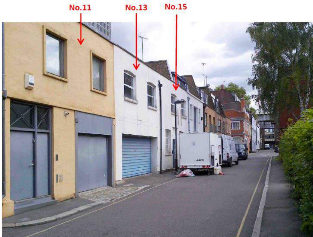
Photo 1: Front elevations of terrace looking south (uphill)
