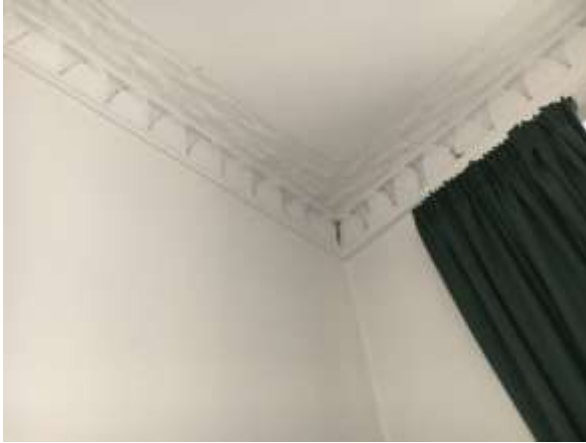
Figure 3.38: Ornate ceiling cornice to front and rear rooms.
