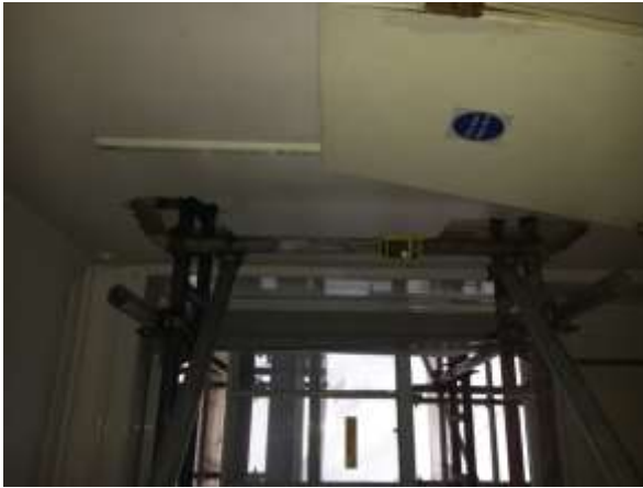
Figure 3.44: Stabilising works to second floor front and showing extant sash.
