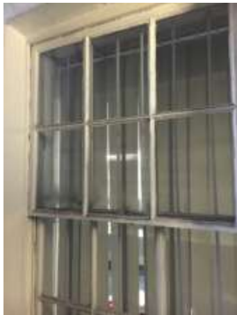
Figure 3.27: Western elevation sash window at lower ground level.
