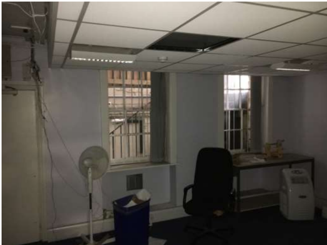
Figure 4.4: Showing suspended ceilings in basement
