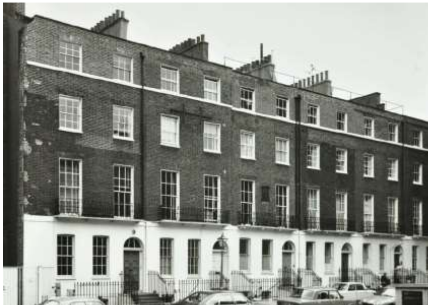
Figure 3.14: Photograph from 1978 showing Nos 27-32 Torrington Square 22 .
