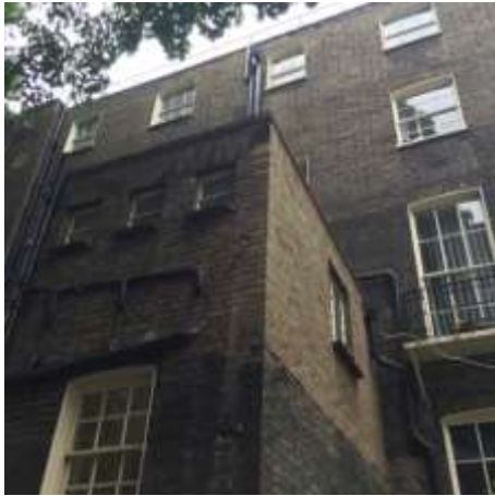
Figure 3.23: Rear elevation to No. 32.
