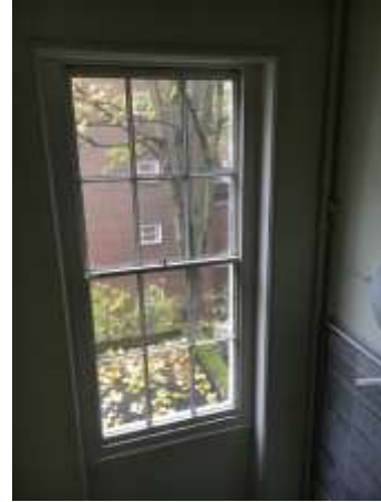
Figure 3.39: Stairlight between first and second floors.
