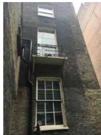
Figure 3.20: Ground to second floor of rear elevation.
