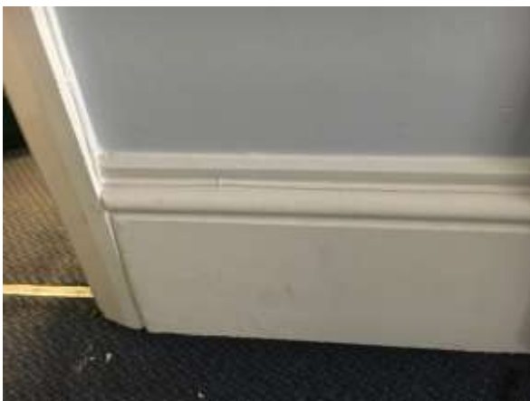
Figure 3.31: Skirting to upper ground floor front room.
