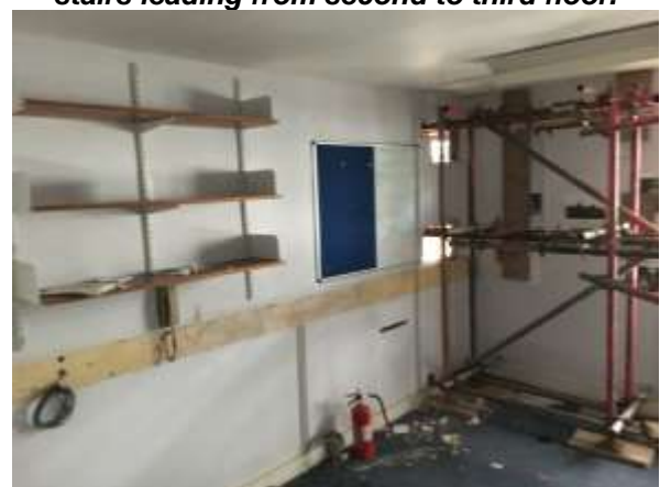
Figure 3.54: Showing the dividing wall between the front rooms at third floor.
