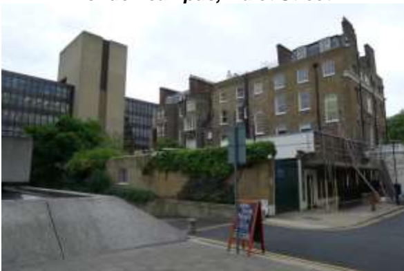
Figure 3.64: Contrast of 19 th century terraces and modern university buildings
