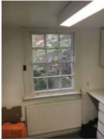
Figure 3.33: Sash window to rear of upper ground floor (northern bay).
