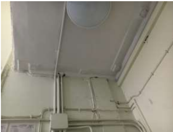
Figure 3.40: Modillioned ceiling to stairwell.
