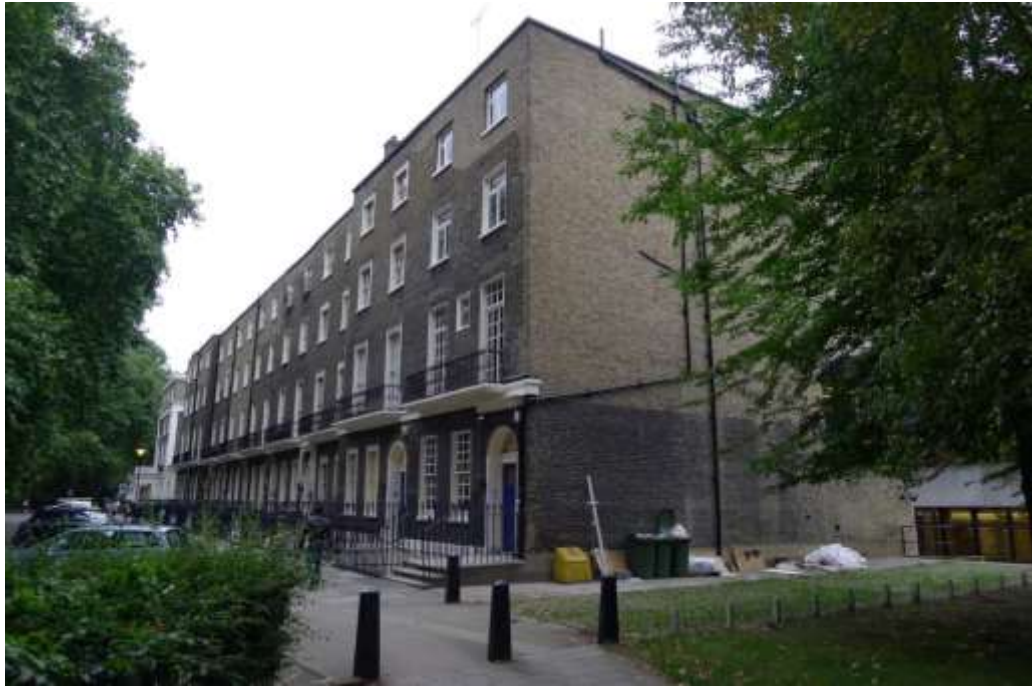
Figure 3.66: Woburn Square (East Side)
