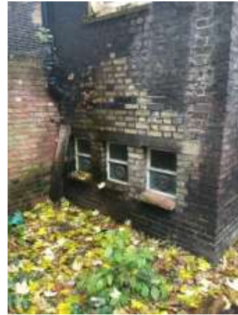
Figure 3.24: Lower ground floor level of closet wing.
