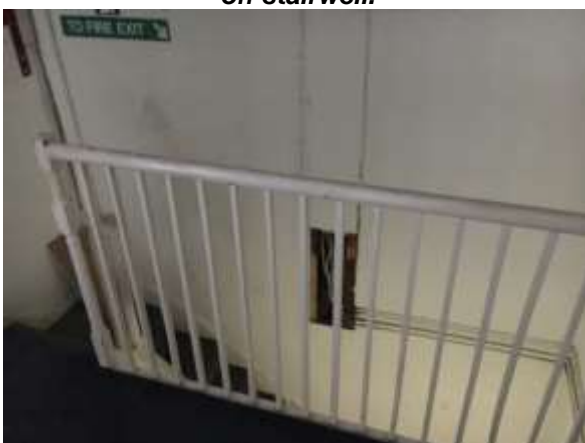
Figure 3.53: Original modest balustrade to stairs leading from second to third floor.
