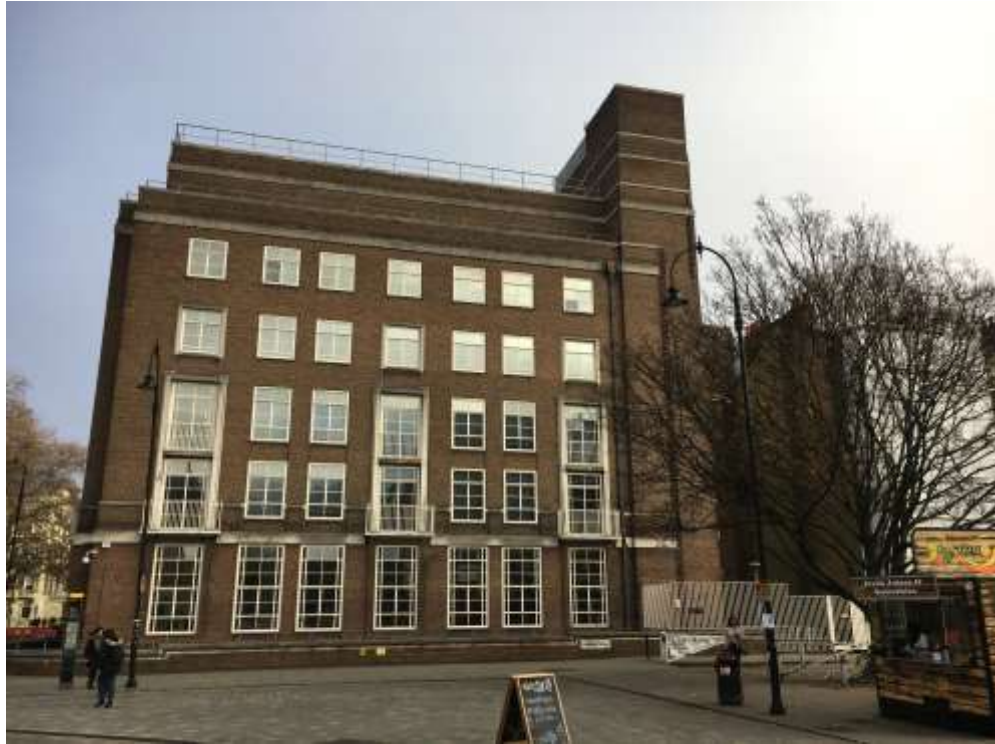
Figure 3.67: Warburg Institute, Torrington Square with the infill site and No. 32 to the right hand side.
