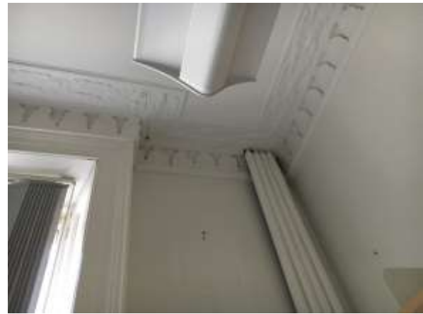
Figure 3.41: Ornate decorative cornicing, sash window and ornate architrave to rear room.
