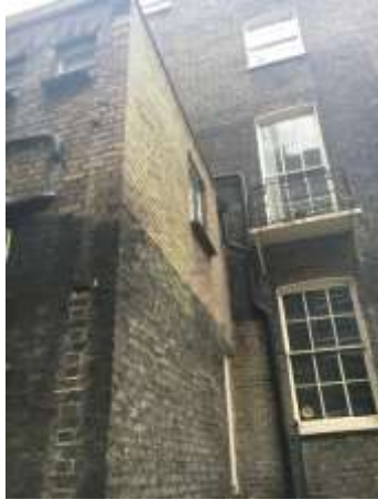
Figure 3.21: Northern elevation to closet wing. Note the mid 20 th century first floor extension.
