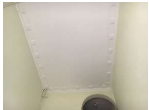
Figure 3.49: Ornate ceiling to staircase leading from first to second floors.
