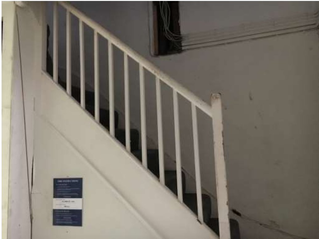
Figure 4.6: Showing existing staircase from second to third floors.
