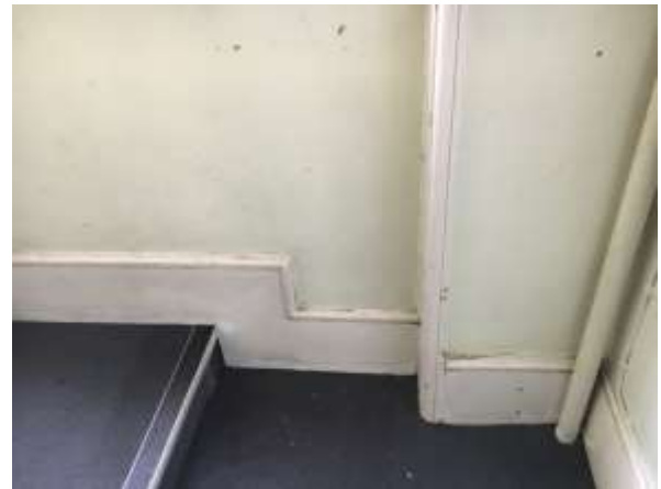
Figure 3.47: Stepped original architrave in stairwell leading from first to second floors.
