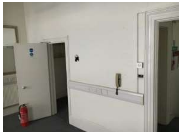
Figure 3.37: Partition wall between the first floor front and rear room (non-original).
