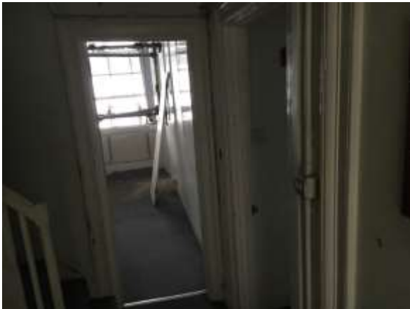
Figure 3.51: Moulded architrave to doorways off stairwell.
