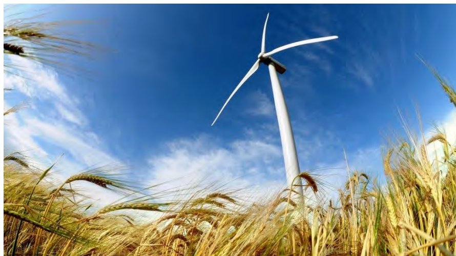
Figure 7. Image of a wind turbine
