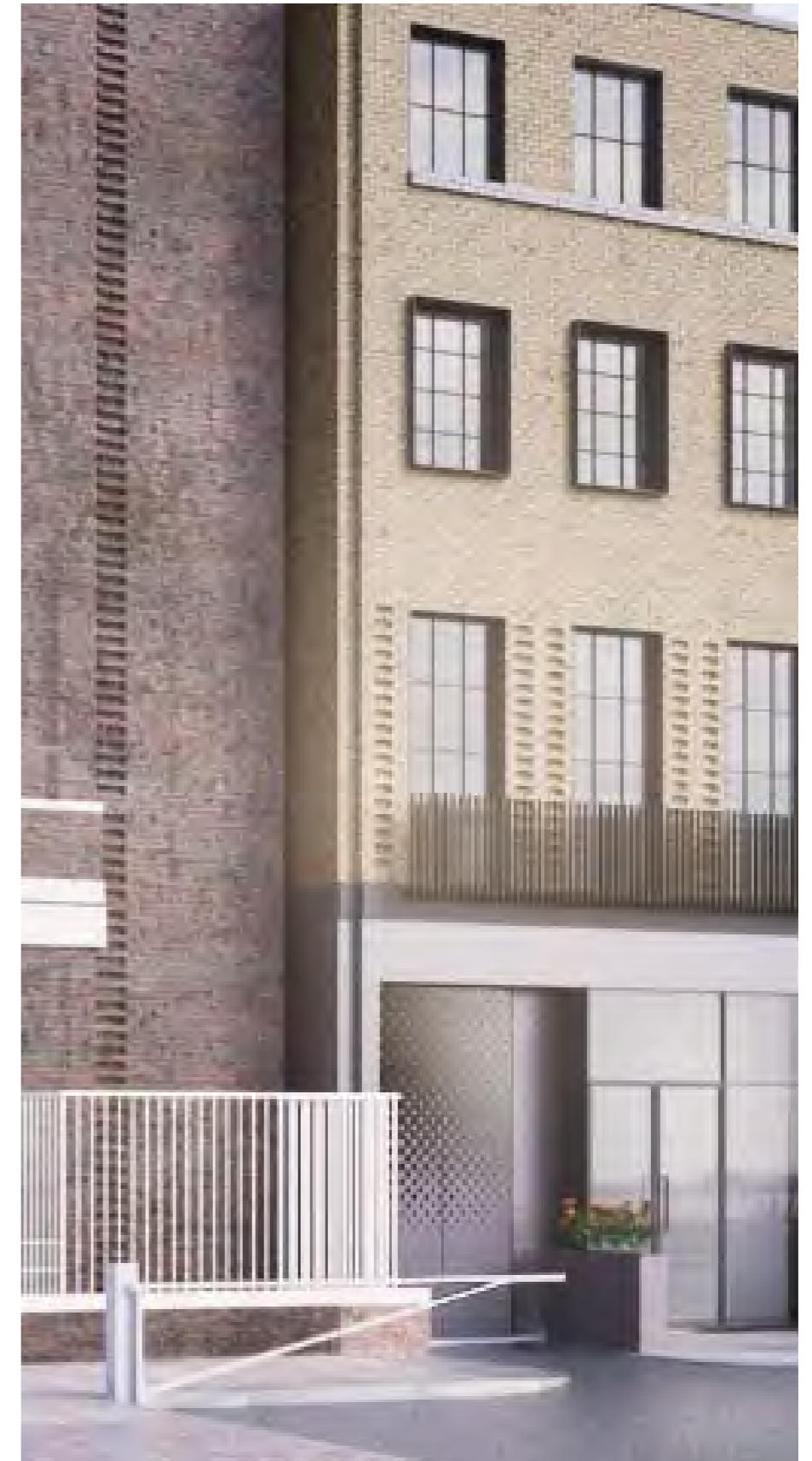
Figure 5.8. Metal gate and road fence by Annex main entrance
