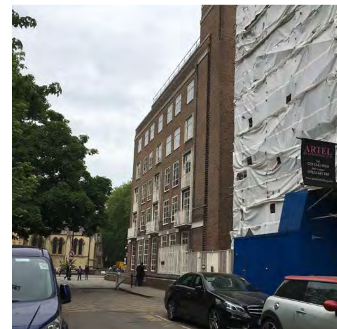
Figure 4.23. Torrington Square gated service access
