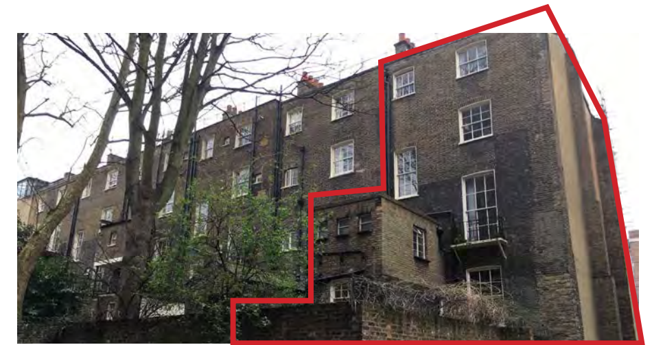
Figure 3.2. No.32 and adjacent terraces back facade
