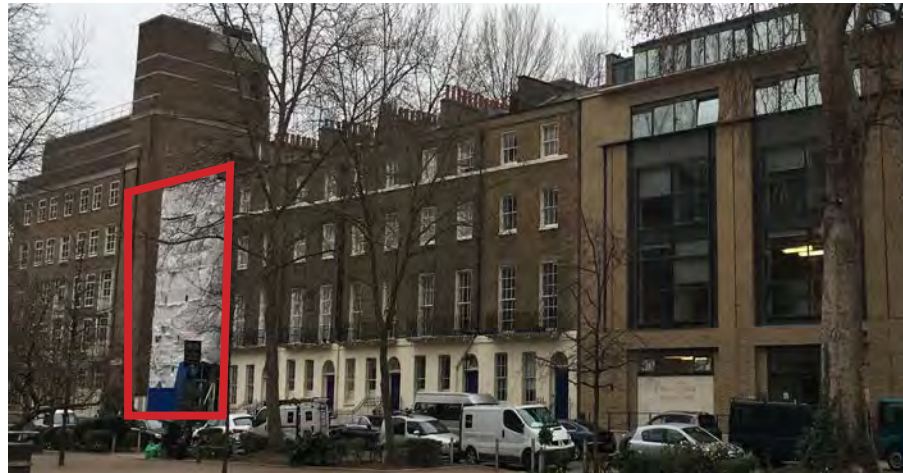
Figure 3.1. No.32 and adjacent terraces front facade
