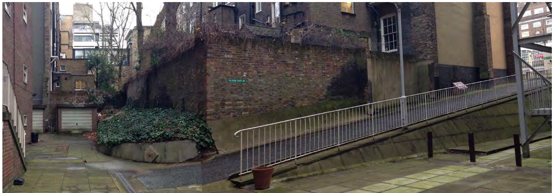
Figure 3.3. Existing ramp access
