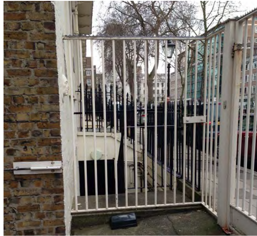
[O] Figure 2.18. Fire exit from basement 32 Torrington Square
