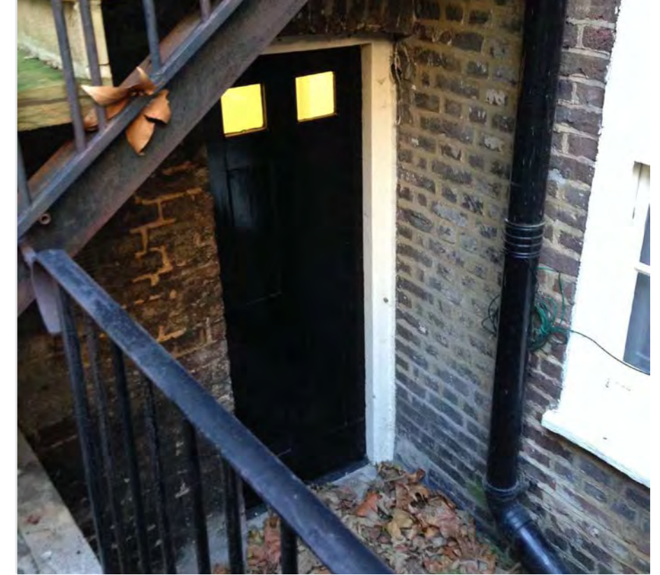
[V] Figure 2.28. 32 Torrington Square Basement garden exit
