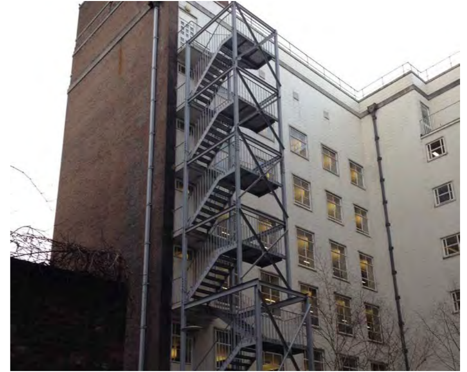
[U] Figure 2.27. Warburg Institute fire exit staircase - view from 32 Torrington Square
