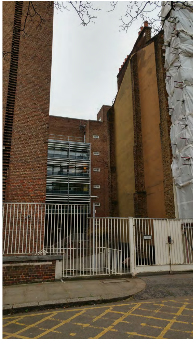
Plate 2: Access ramp section of the site with metal access gates.
