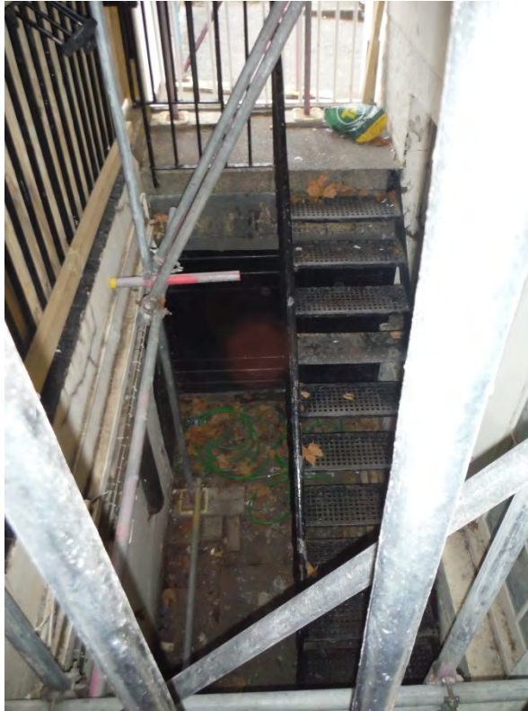
Plate 5: Light well at south western corner of the site.
