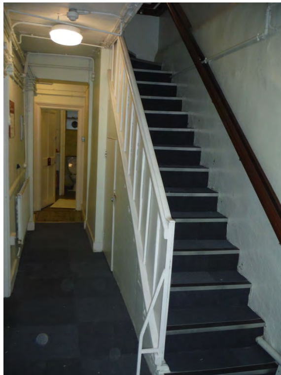
Plate 8: Stairwell down to the basement.
