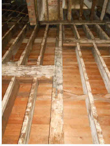
P 48 Second Floor – Area S7
