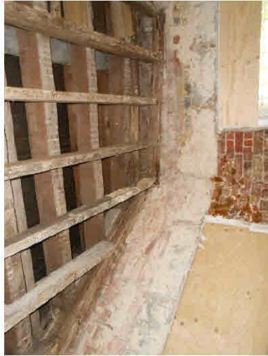
P 46 Second Floor – Area S2
