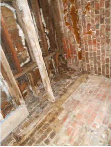
P 44 Second Floor – Area S2
