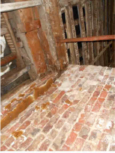
P 45 Second Floor – Area S2
