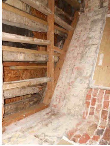
P 47 Second Floor - Area S2
