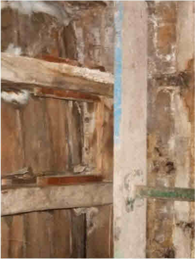
P 43 Second Floor – Area S2
