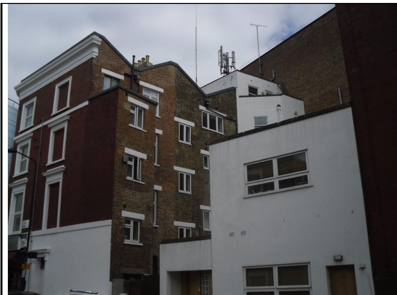
View from Cliff Road - Rear of application site & neighbouring buildings – 149 – 151 York Way
