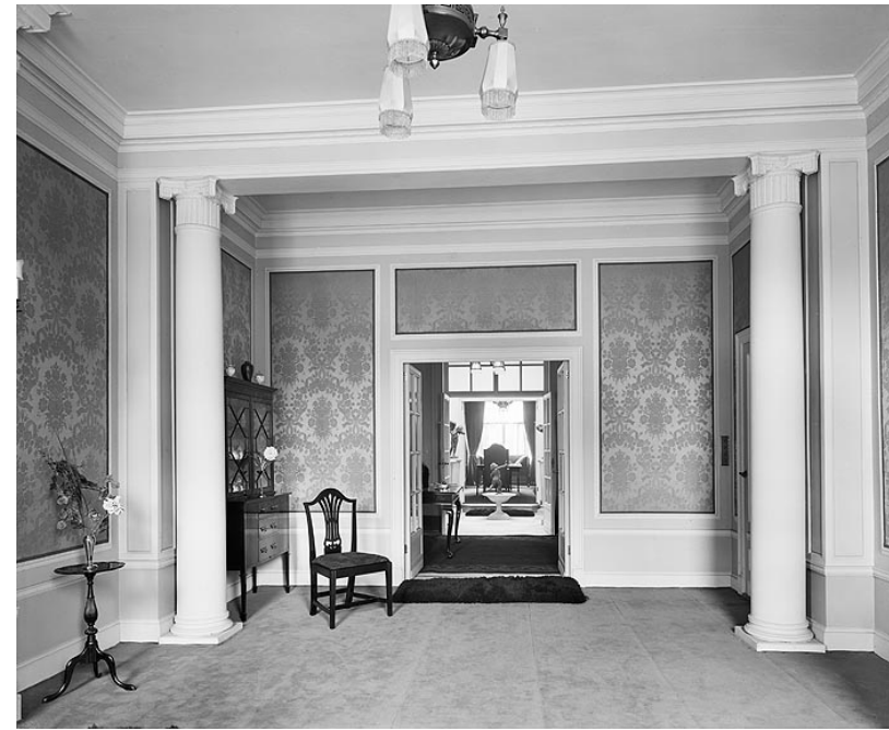
PHOTOGRAPH OF THE MORNING ROOM (FRONT GROUND FLOOR) No 14 CHESTER TERRACE, 1915, ILLUSTRATING THE USE OF COLUMNS TO SEPARATE THE FRONT ROOM. HISTORIC ENGLAND ARCHIVE.
