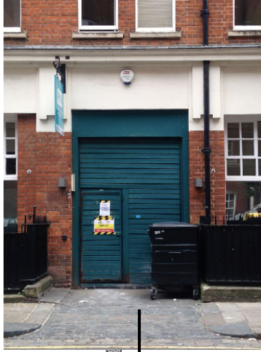
Existing shutter to be replaced
