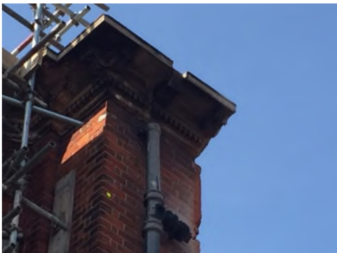
Existing retained chimney and coping details
