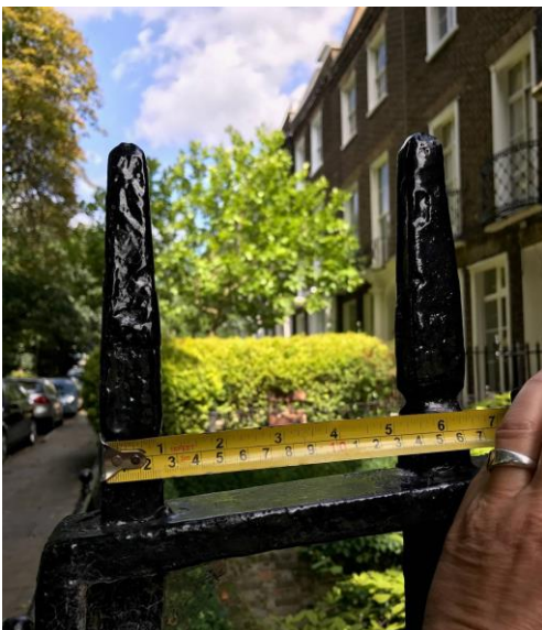
Figure 3: Grove Terrace railing head
