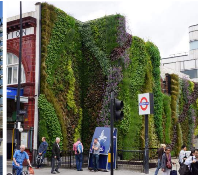
Edgware Road Tube Station, London Installed November 2011
