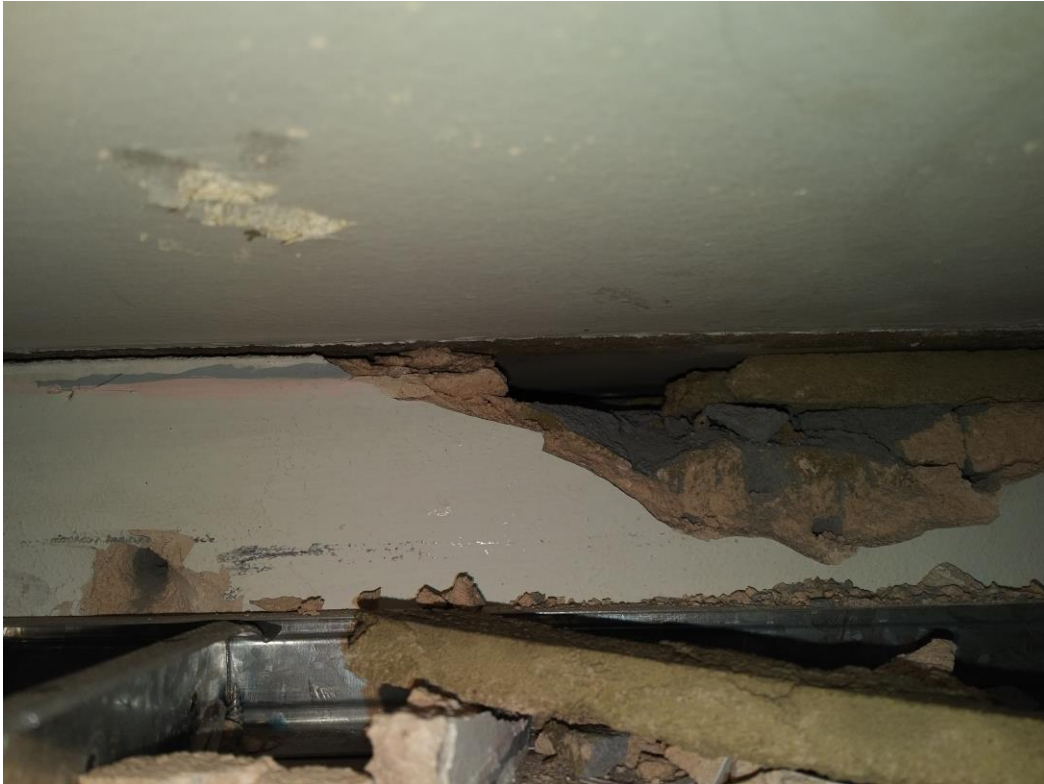
Figure 1: Top of partition wall at lining removal
