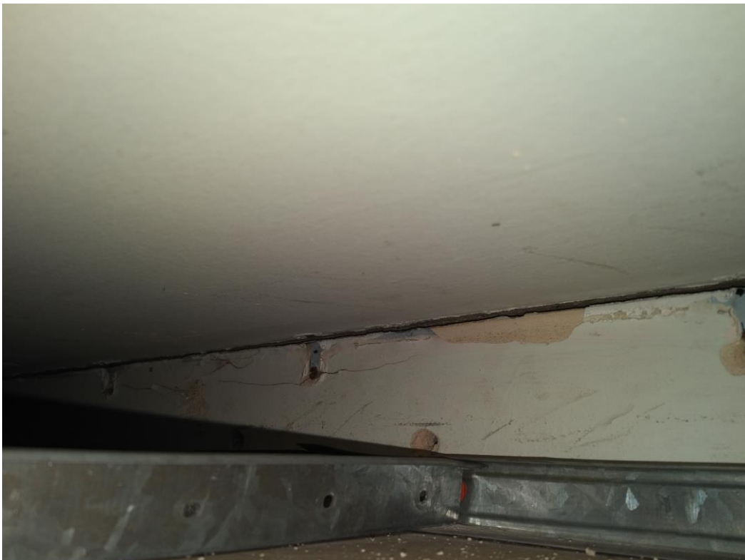
Figure 2: View along partition wall in ceiling void
