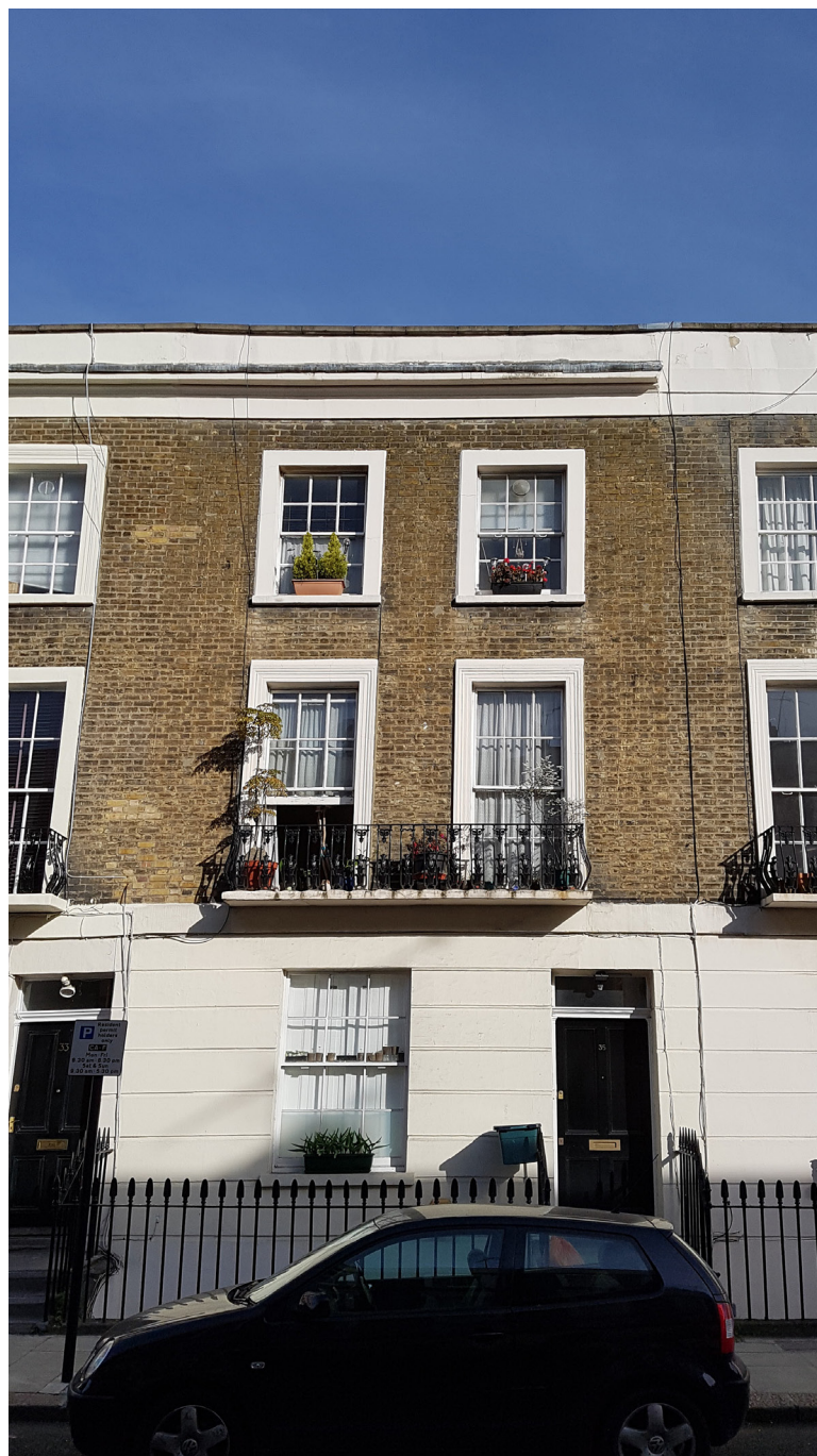
Figure 10/ Front facade of 35 Greenland Road
