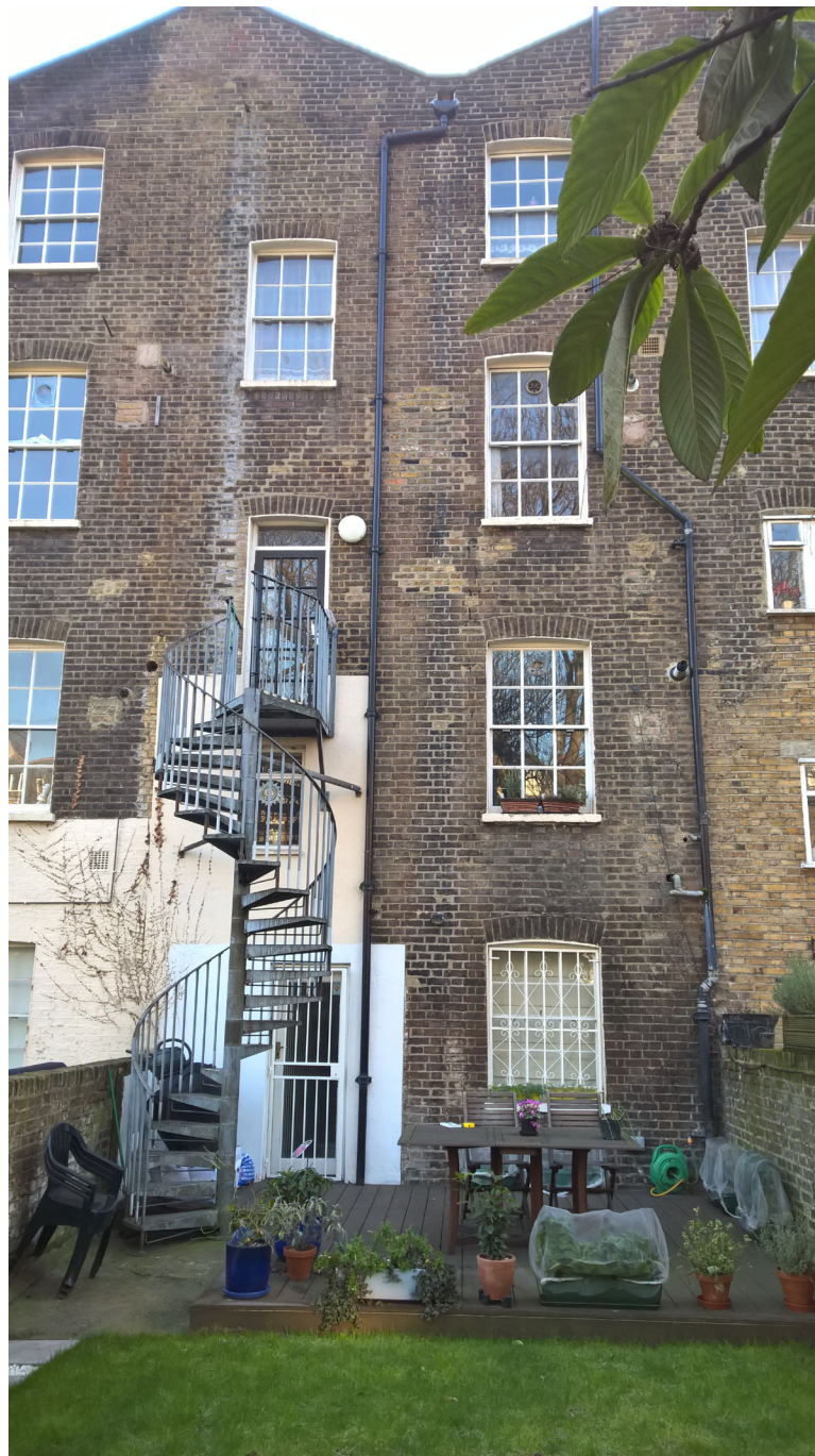
Figure 11/ Rear facade of 35 Greenland Road
