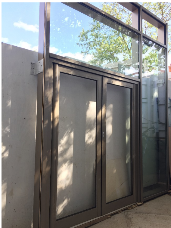
Curtain walling ED-51, elevation and detail: Doors with fixed glazed side- and over-panel; side panel
